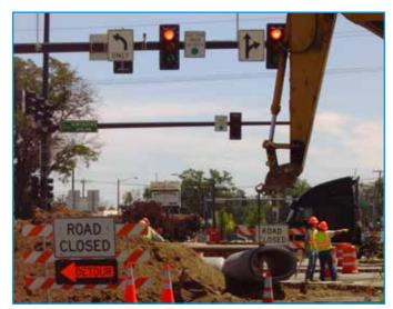
The US 85/US 34 bypass reconstruction in Greeley will improve safety and accommodate increasing traffic. CDOT crews removed and replaced pavement, medians, shoulders, and traffic signals in addition to extending and widening turn lanes. Projects like this help us get more out of the existing transportation system.
