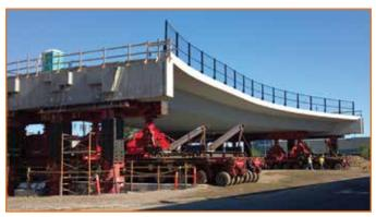
This new bridge over I-70 at Pecos was built and slid into place, reducing disruption to traffic on I-70 and saving construction costs.
