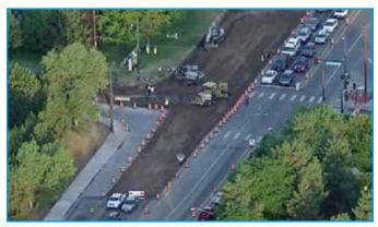
Taken just before the morning rush hour, this photo of Colorado Boulevard and Hampden Avenue resurfacing highlights the large work areas that are possible with an aggressive phasing approach (17 days). CDOT received positive feedback for the quick work at this congested city intersection.
