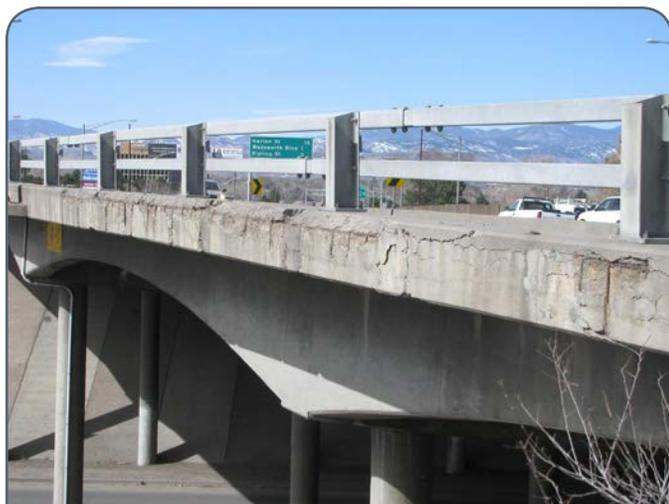
Work on this bridge over I-70 at Sheridan and Tennyson in Denver included concrete crack repair with epoxy injection; girder strengthening with composite fiber wrap; and substructure column repairs.
