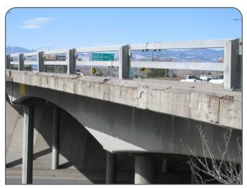
Work on this bridge over I-70 at Sheridan and Tennyson in Denver included concrete crack repair with epoxy injection; girder strengthening with composite fiber wrap; and substructure column repairs.
