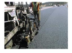
rubber. To ensure the highest quality, the placement temperatures must be 65 degrees and rising. This makes night paving in Colorado virtually impossible. Since traffic congestion requires most construction in Colorado, especially in urban areas such as Denver and Colorado Springs, to be conducted at night, there is a very small window of opportunity to pave.
