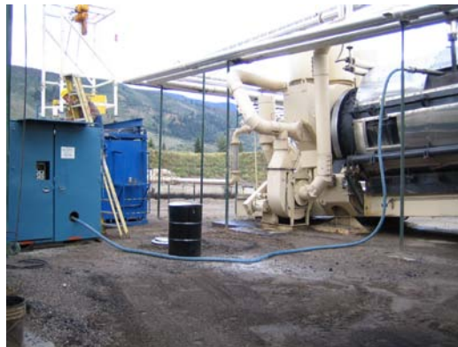
Figure 8 Feeding Sasobit through Fiber Feed Line
