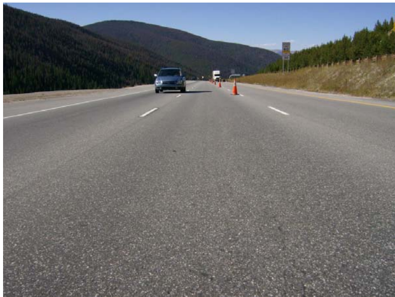
Figure 17 Overall Surface Texture of HMA Control and WMA Test Sections: Excellent Performance
