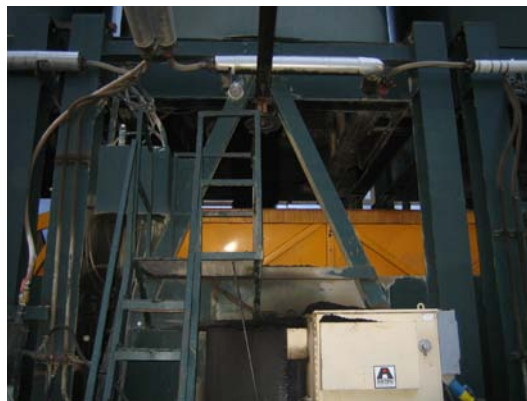
Figure 9 No Visible Smoke or Fumes from Sasobit WMA Production at the Plant
