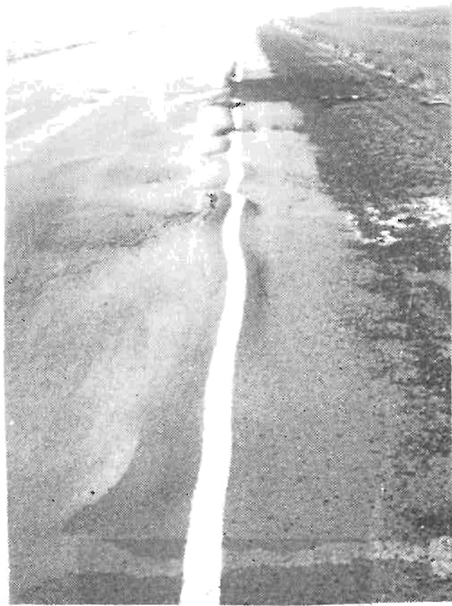
Fig. 3. The Surface of a Pavement Requiring "Complete Rehabilitation" in 12 Months.
