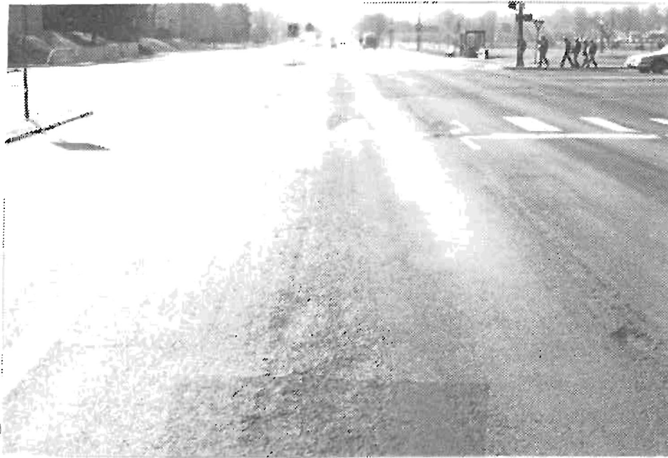
Fig. 1. A "High Maintenance" Mix Experiencing Raveling After 15 Months.
