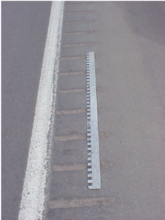
Figure A-1. At Eagle on I 70 eastbound , CDOT constructed nine rumble strip configurations. This figure shows the spacing of the grooves in section 1 – the first section at the west end of the test sections. The black and white squares on the straight edge are one inch on a side. The straight edge shows that the grooves are 2” wide with 10” flats in between. This spacing was ground for 1000 feet in a continuous configuration and then for another 1000 feet in an interrupted configuration – 12 feet of grooves and 6 feet without grooves.
