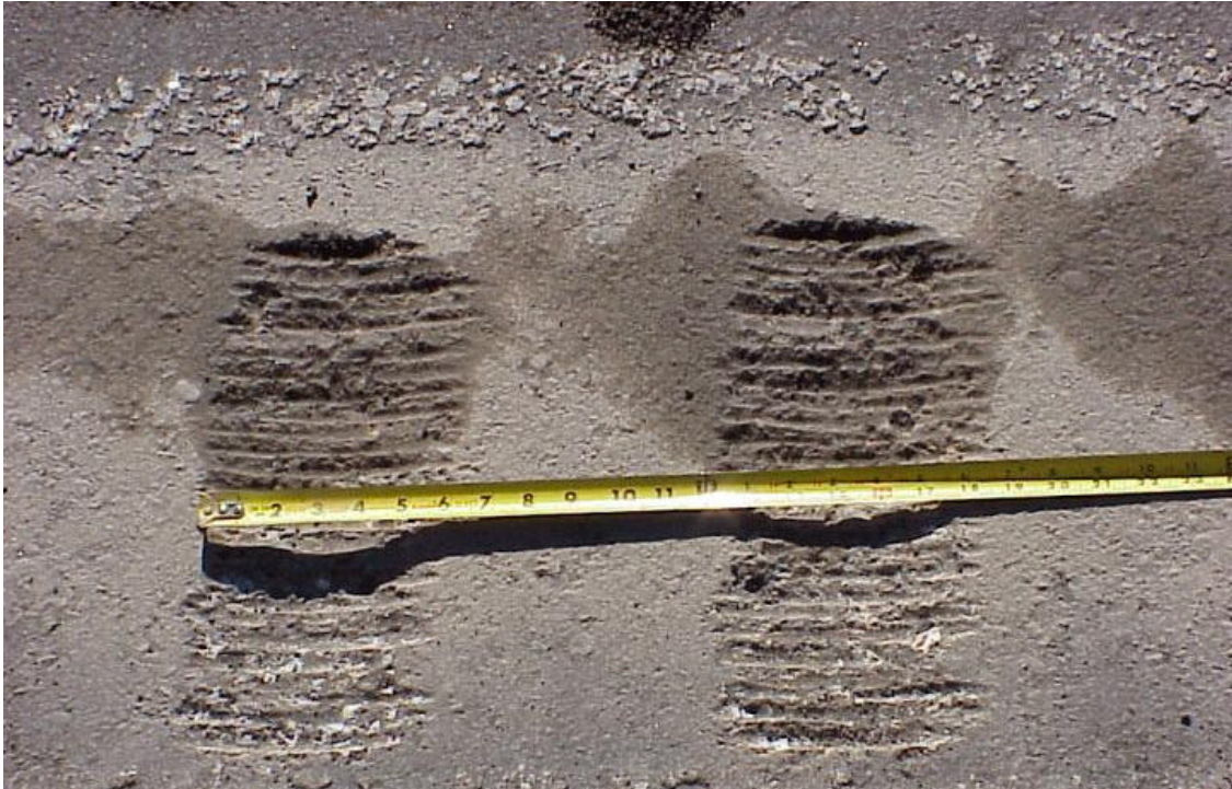
Figure 5. One of the shallower sections of standard rumble strip. The grooves are on 12-inch centers. The wear on the grinder teeth is shown by the uneven shape and variation in depth along the grooves.
