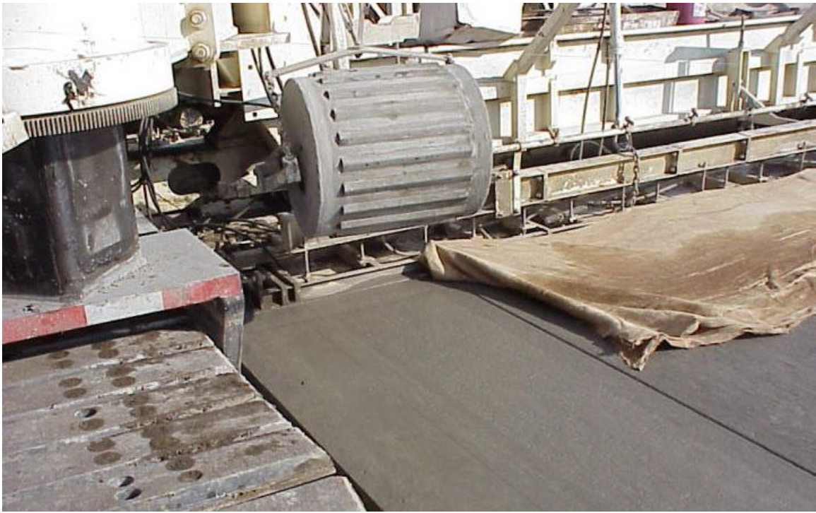
Figure 15. The roller that forms rumble strips in new concrete pavement. The roller has been raised because the paving operation is approaching an intersection. This roller forms rumble strips on the left shoulder.
