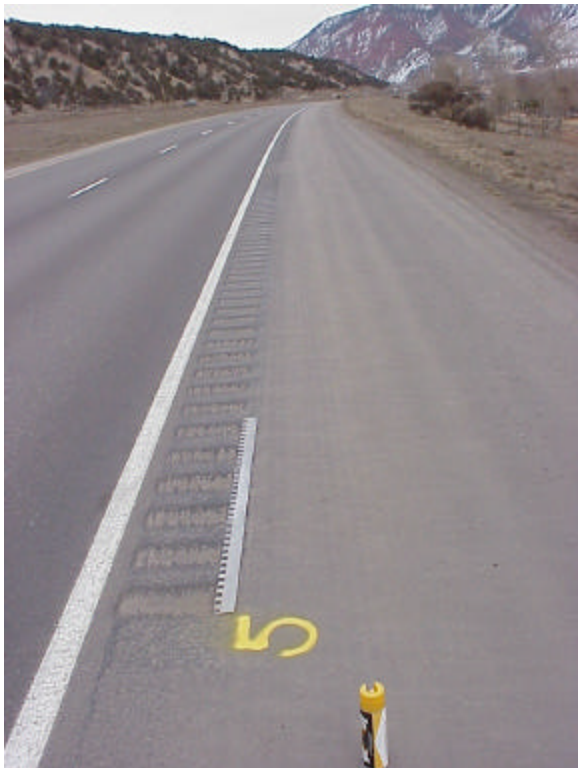
Figure A-14. Section 5 was ground in an interrupted pattern. The old standard style rumble strip has 12 foot gaps after 48 feet of rumble strip. The white arrow points to a gap in the rumble strip.
