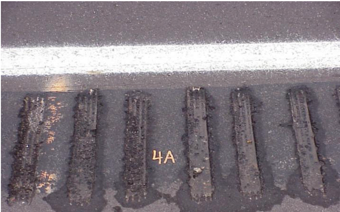
Figure 14. Test section 4A on I 70 at Eagle - 2" groove 3" flat. This picture shows how the rumble strip may capture water and debris. The slight variations in the groove spacing are caused by the spacers used on the grinding drum.
