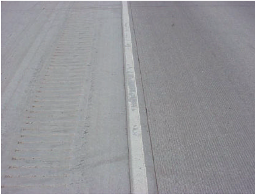
Figure A-19. The concrete rolled-in rumble strip used for the study was placed away from the shoulder stripe at the request of CDOT maintenance.
