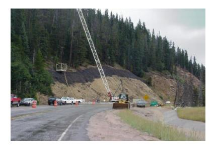
Figure 1. Lifting materials to the top of the slope.
