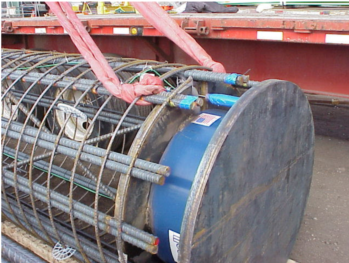
Figure 3.1. Photo of the O-Cell Placed in the Broadway Test Shaft
