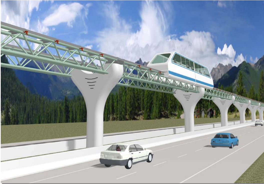
Figure 39: Concept C - Rendering of Steel Truss Guideway
