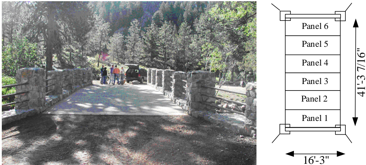
Figure 13. The bridge in O’Fallon Park, Denver, Colorado
