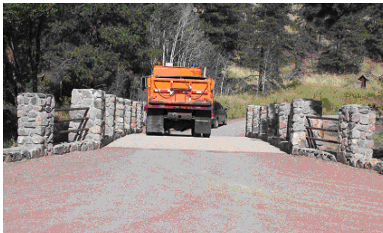
(b) Back view of the loading truck
