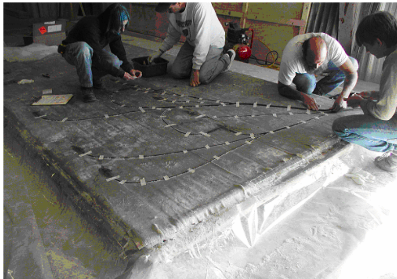
Figure 15. Installation of fiber optic sensors in the FRPH panel
