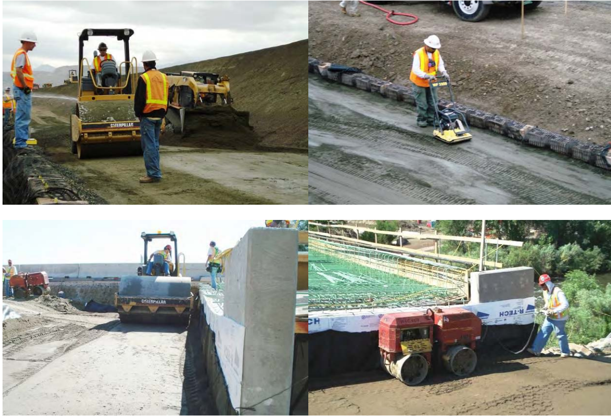
Figure 4-6. Near Wall Compaction Techniques
