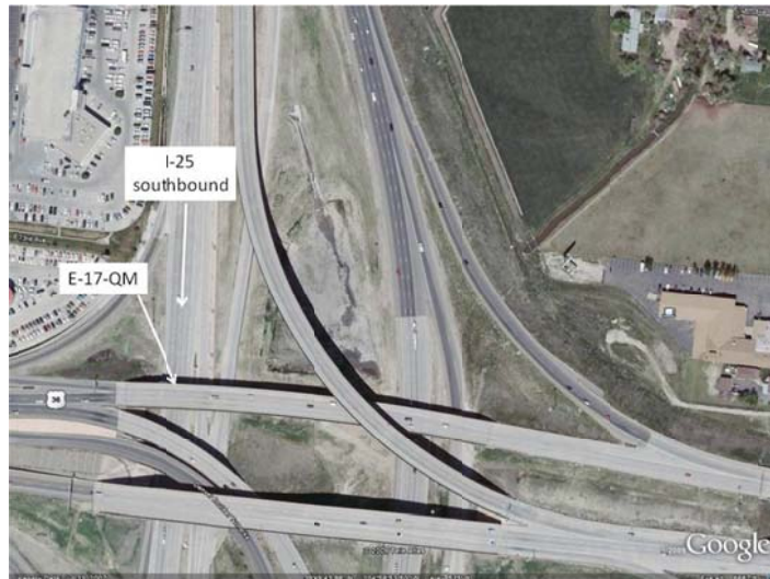
Fig 3.1 Bird's eye view on Bridge E-17-QM
