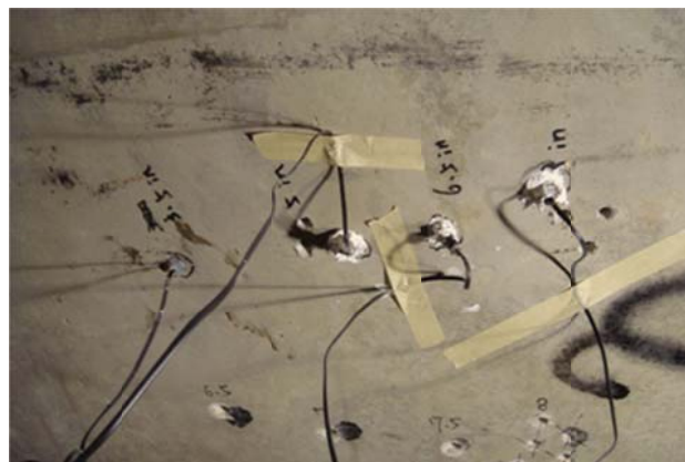
Fig 3.14 Integrated sensors installed in the deck.
