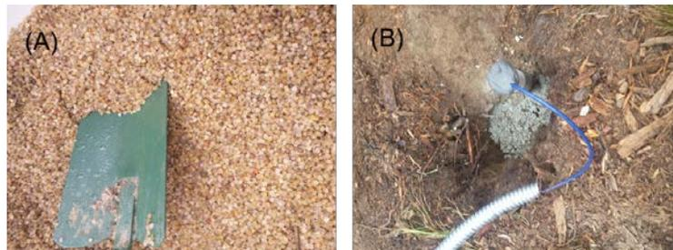
**Figure C.13 Piezometer installation (a) coarse sand used for filter, (b) borehole sealed with bentonite**
