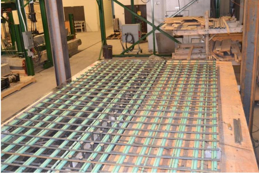
**Figure 53 - Slab Reinforcing Placement**
