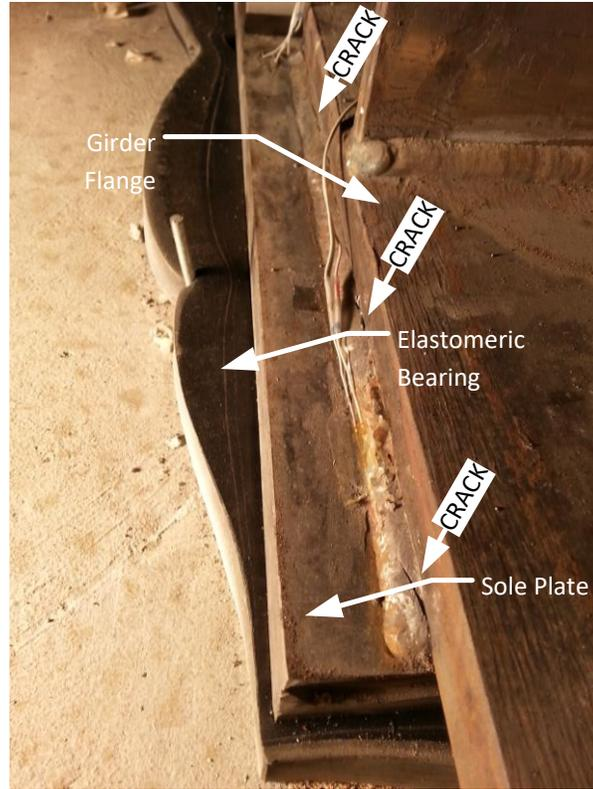
**Figure 68 - Failed Weld on East Side of North Girder**
