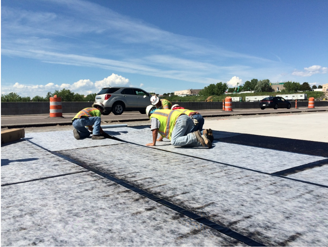
Figure 4-6. Installation of Protecto Wrap waterproof membrane
