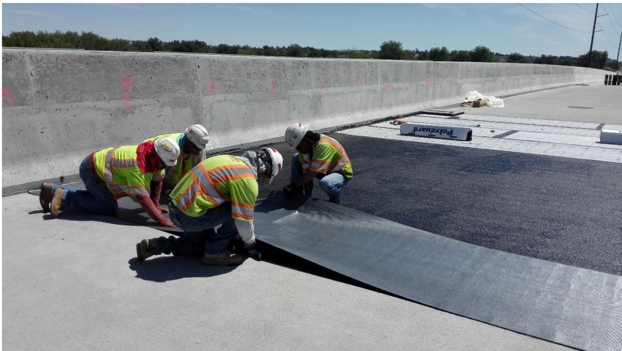
Figure 4-7. Installation of Polyguard waterproof membrane
