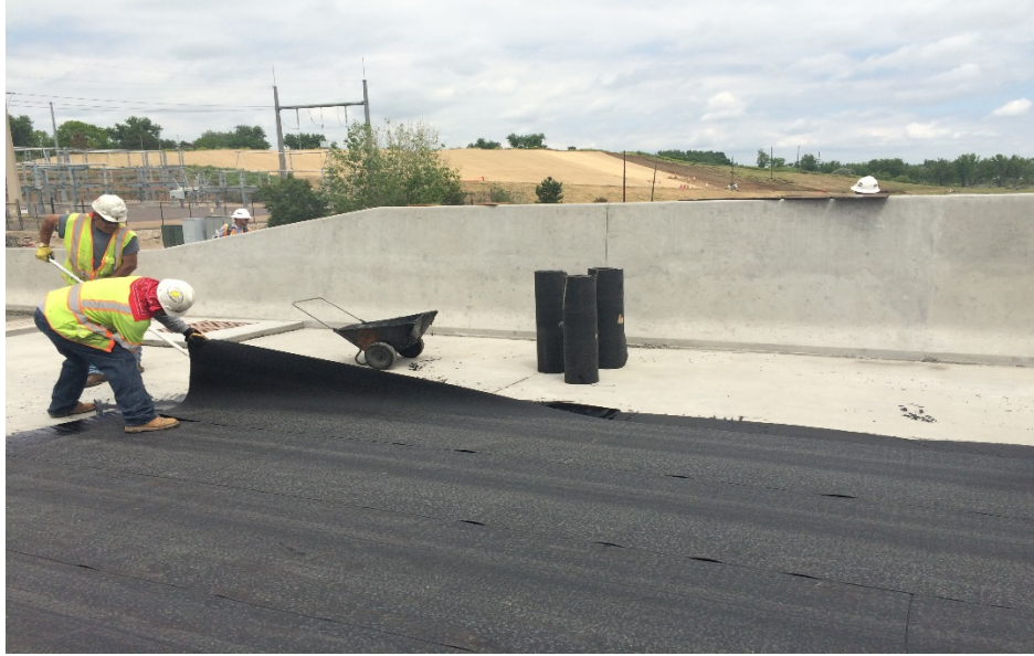
Figure 4-10. Installation of hot mix control section
