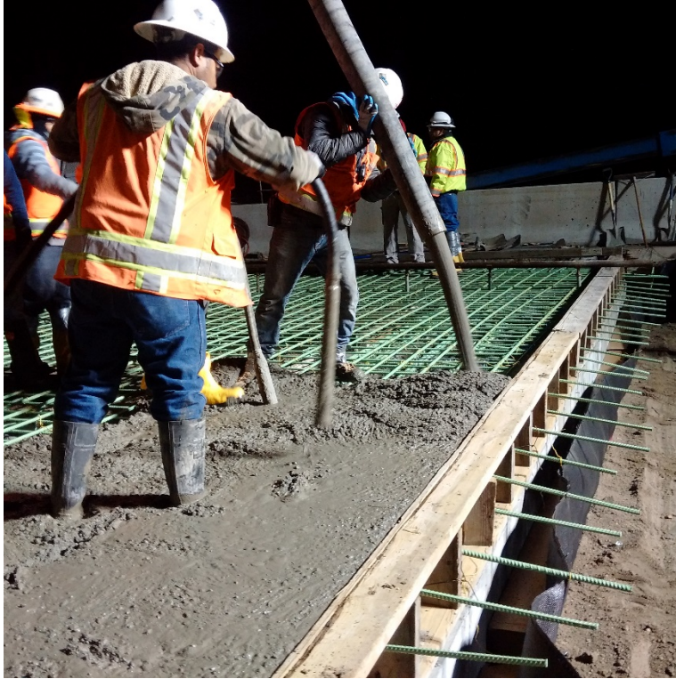
Figure 4-4. Concrete casting
