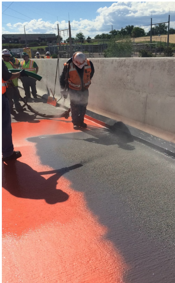
Figure 4-9. Installation of Bridge Preservation™ waterproof membrane
