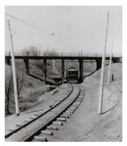
Figure 164. D&SP streetcar in Slaughterhouse Gulch, c.1910. Note the poles carrying the electric lines installed at an angle outward to keep the electric lines taught.<sup>710</sup> (Image from the Collection of the Littleton Museum. May not be reproduced in any form without permission of the Littleton Museum.)
