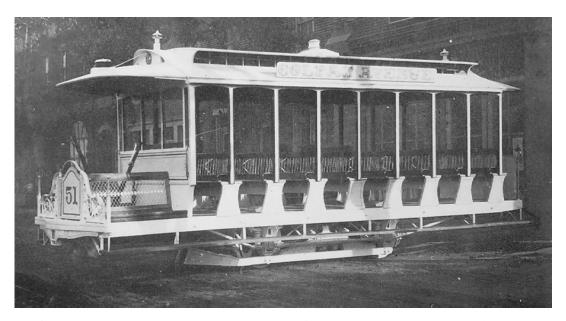
Figure 9. A Denver Tramway open cable car, which would have been used in good weather.
