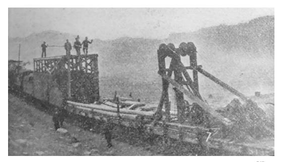
Figure 115. Crews stringing wire during the construction of the D&I.547
