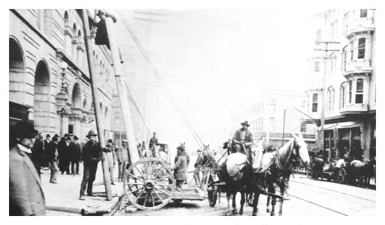
Figure 60. Erecting poles at the corner of 17th and Stout Streets for the conversion to electric traction.<sup>310</sup>
