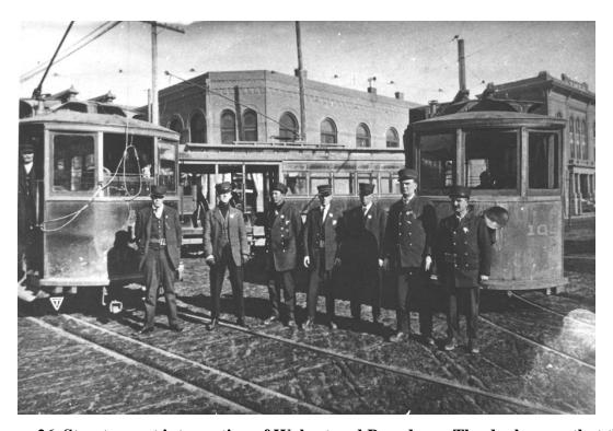
Figure 26. Streetcars at intersection of Walnut and Broadway. The dual gauge that the interurban shared with the streetcar is visible.<sup>202</sup>
