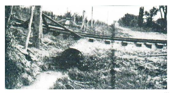
Figure 148. A corrugated culvert on the GJ&GRV interurban line to Fruita. 666
