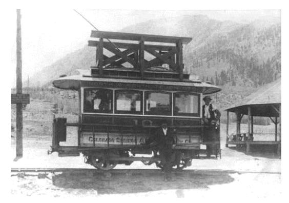
Figure 29. Horsecar operated by the CS&M, later repurposed for electric service, c.1900.<sup>211</sup>
