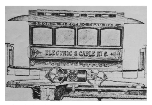
Figure 55. Graphic of Short's electric motor and conduit underneath the streetcar. <sup>287</sup>
