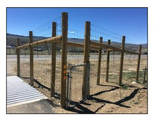
Figure 7-4. Pedestrian access point outfitted with a swing gate.
