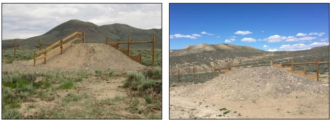
Figure 2-2. Example of an escape ramp with a 2:1 slope with perpendicular rail fence (left) and a ramp with a 3:1 slope without rail fence (right).
