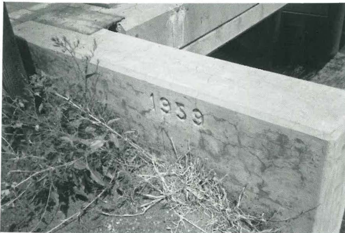
PICTURE #5 STRUCTURE D-20-AC MAP CRACKING IN CURB
