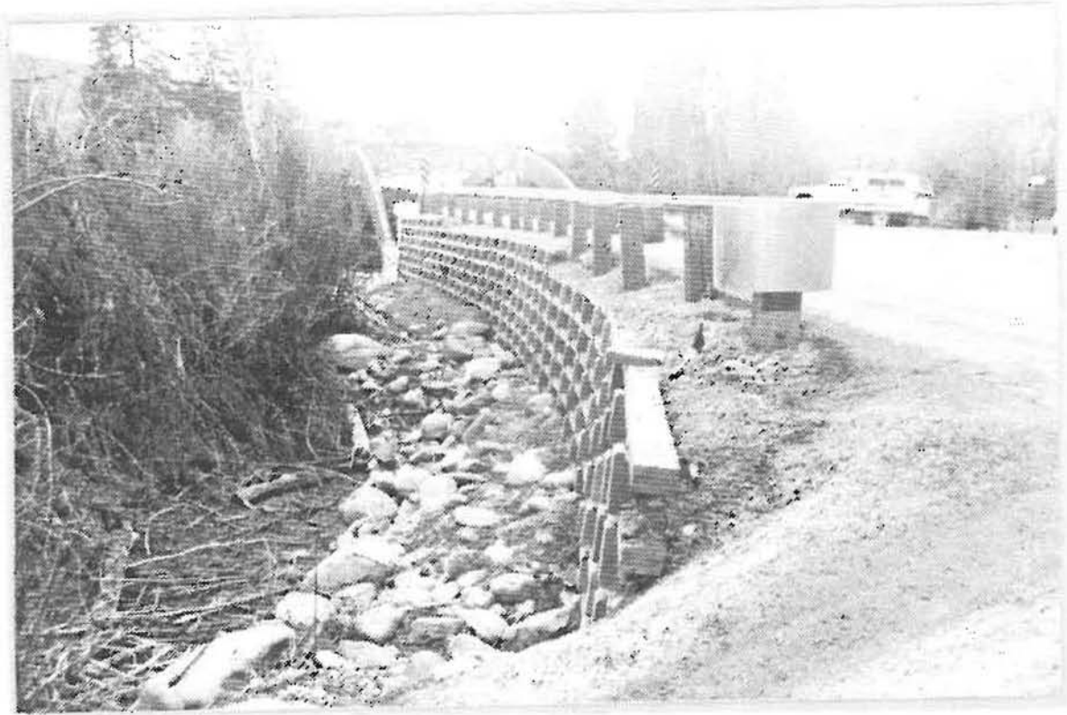
Figure 14. completed east cribwall
