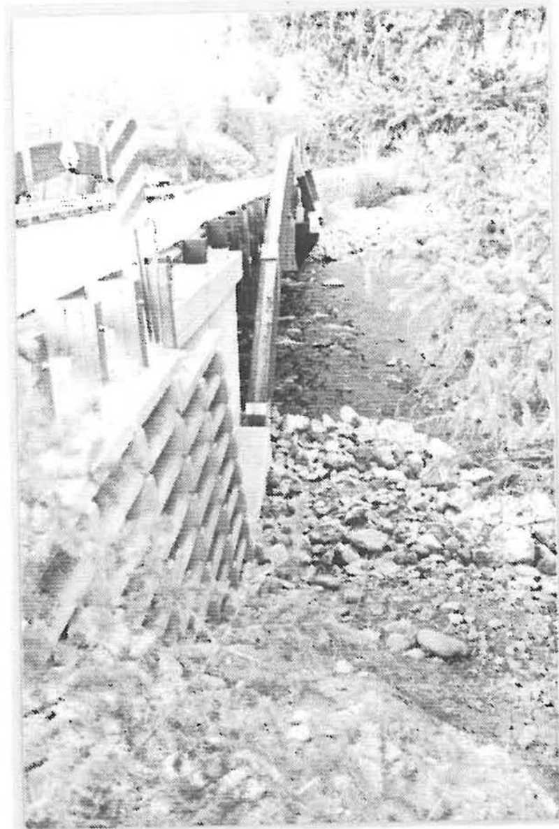
Figure 16 view of the completed structures on project BRO 0057(2)
