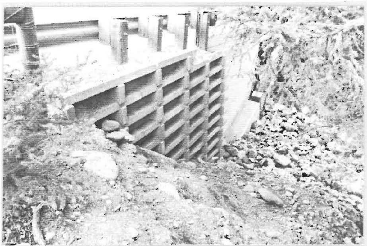
Figure 15. completed west cribwall
