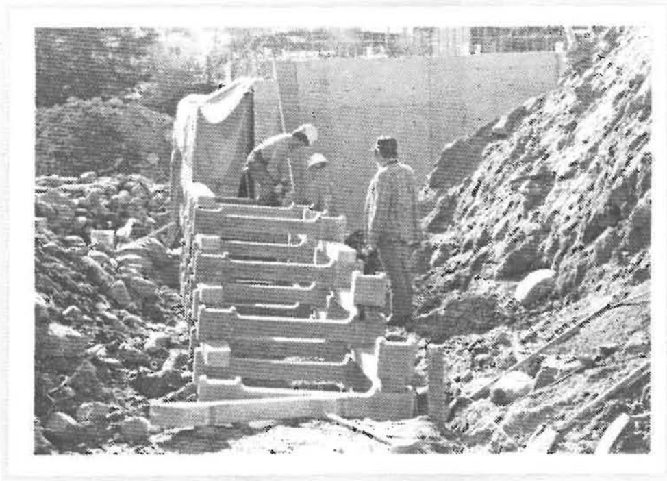
Figure 9. Close-up view of the concrete cribwall components
