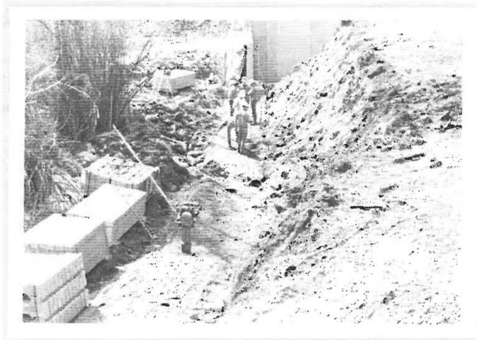
Figure 6. Foundation preparation for the east wall
