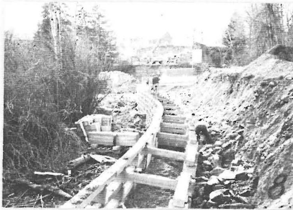
Figure 12 progress of the east cribwall
