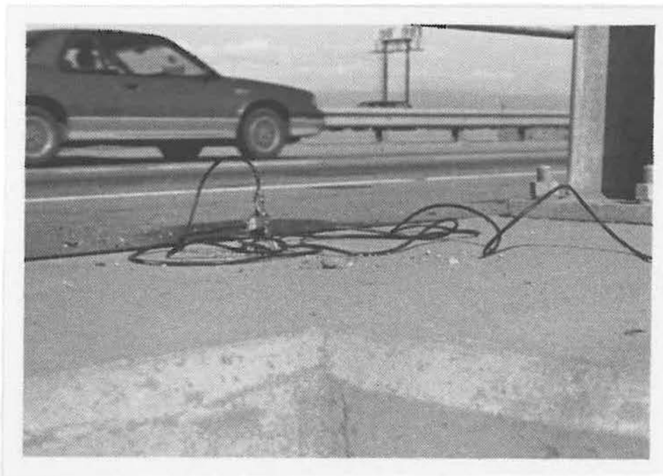
Photograph 2. A ground was secured to complete the circuit.
