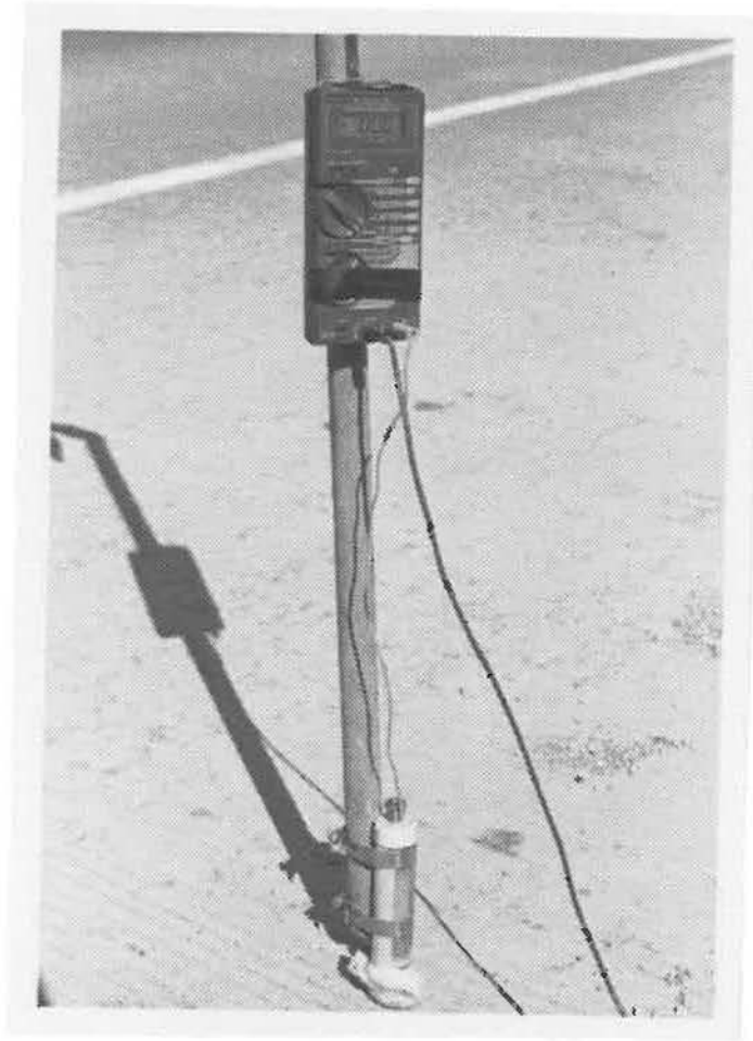
Photograph 5. Copper-copper sulfate half-cell is used on bare decks. Voltages are recorded.
