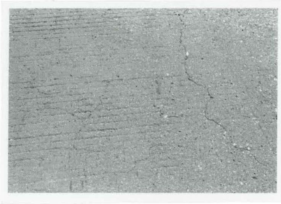
Photograph 7. Surface detail of deck C-17-AT. April, 1990. Low slump concrete with fly ash.
