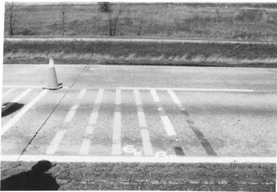
Photo 23. 3/29/88 3M removable grade preformed plastic on concrete.
