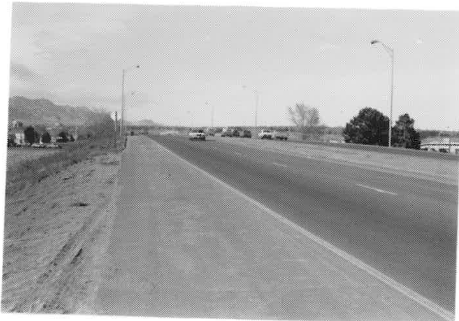
Photo 9. 1/25/88 I25 southbound, milepost 138, Harrison Road Interchange, 1986 epoxy paint.
