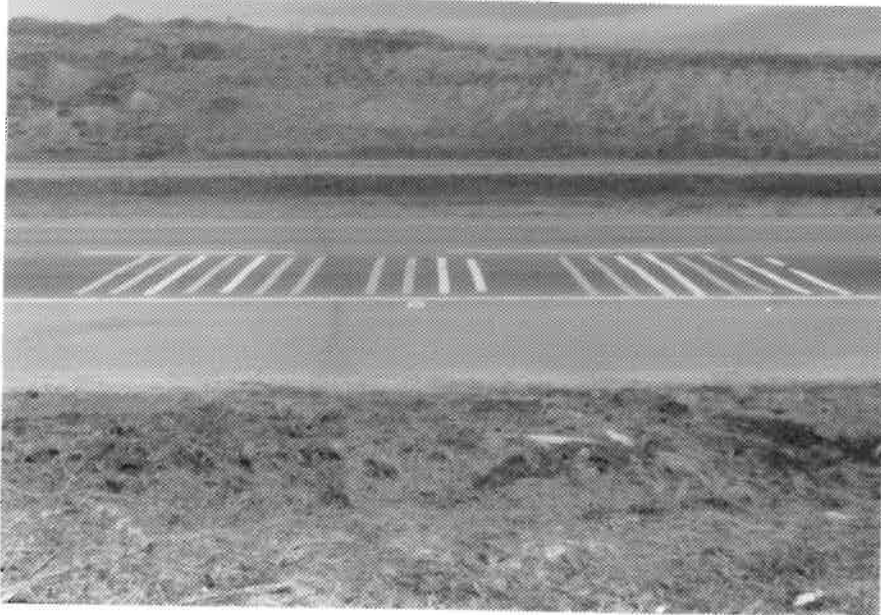
Photo 29. 3/29/88 Prismo removable grade preformed plastic on asphalt.
