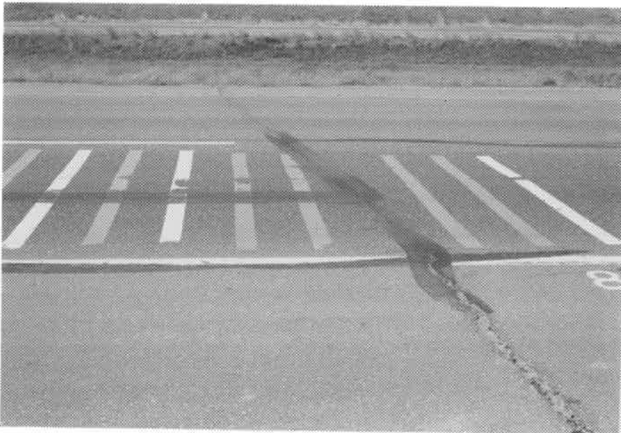
Photo 48. 3/8/89 Prismo permanent grade preformed plastic on asphalt.
