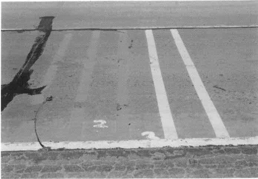
Photo 34. 3/8/89 Volare permanent grade preformed plastic on concrete.
