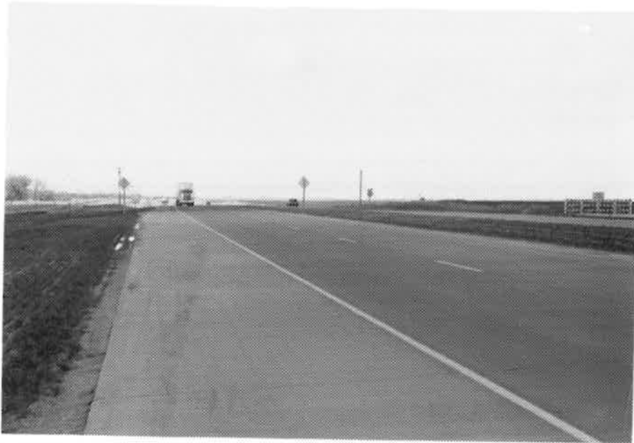
Photo 10. 4/13/87 I76 southbound, just south of Bromley Lane, 1986 epoxy paint.
