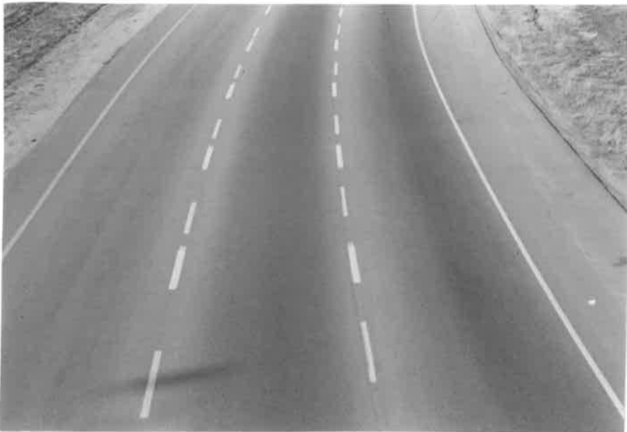
Photo 4. 12/84 I70 westbound, milepost 248, near El Rancho Interchange, 1984 polyester paint installed.
