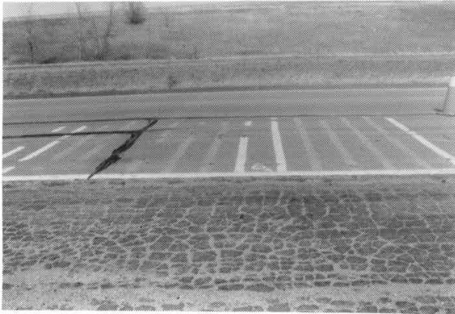
Photo 37. 3/8/89 Prismo permanent grade preformed plastic on concrete.
