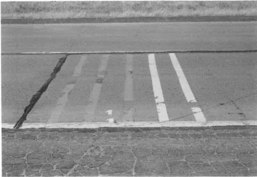
Photo 31. 3/8/89 Pavemark permanent grade preformed plastic on concrete.
