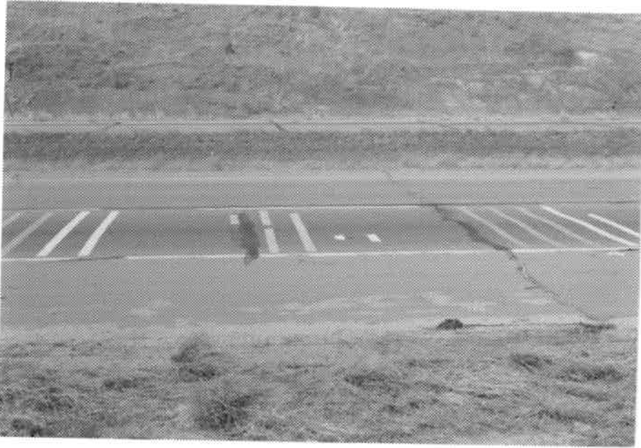
Photo 43. 3/8/89 Seibulite permanent grade preformed plastic on asphalt. (Far left four stripes)
