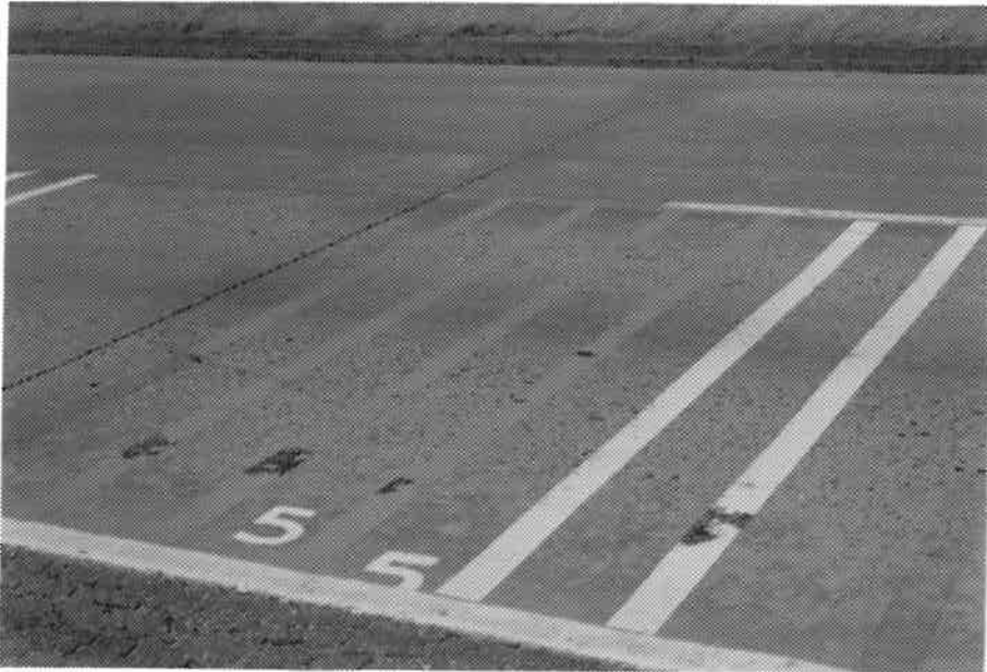
Photo 25. 3/29/88 PB Laminations removable grade preformed plastic on concrete.
