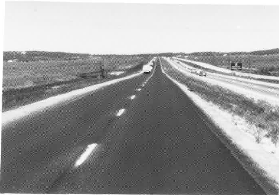
Photo 1. 6/28/84 I25 southbound, milepost 159, north of Monument, 1984 epoxy paint.
