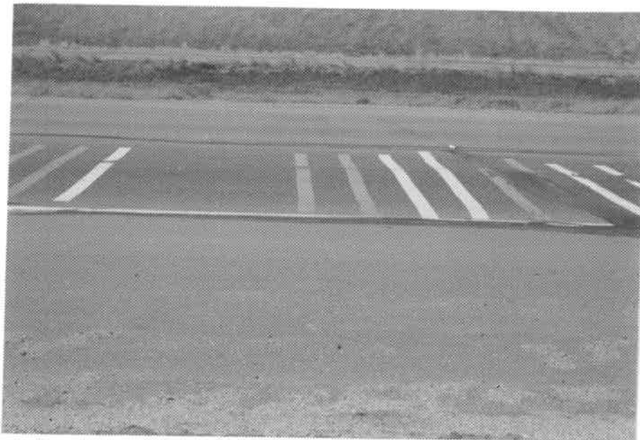
Photo 49. 3/8/89 Prismo permanent grade preformed plastic on asphalt.
