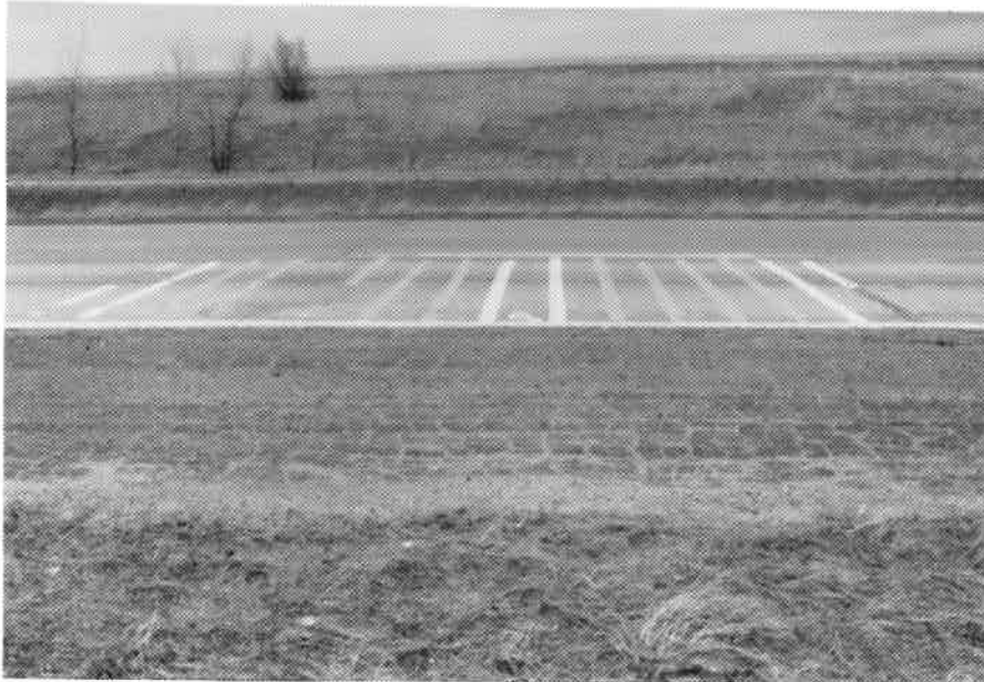
Photo 24. 3/29/88 Prismo removable grade preformed plastic on concrete.
