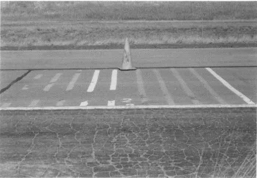
Photo 32. 3/8/89 Swarolite permanent grade preformed plastic on concrete.
