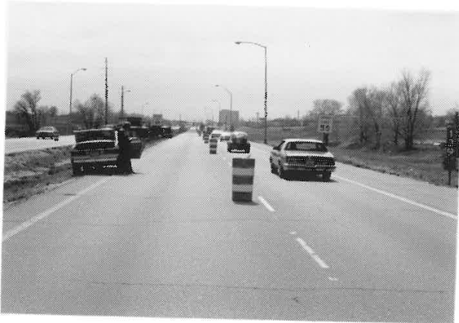
Photo 7. 4/17/89 I25 southbound, milepost 139, 1985 and 1988 epoxy paint.
