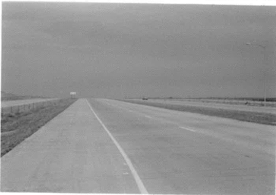
Photo 14. 2/27/89 I76 southbound, just north of Bromley Lane, 1986 epoxy paint overstriped with fast-dry alkyd paint.
