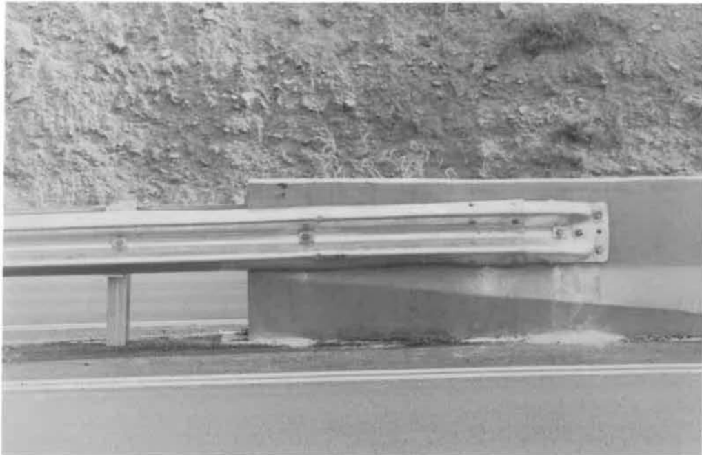
Photo B4. Brakemaster transition section fastened to concrete barrier.
