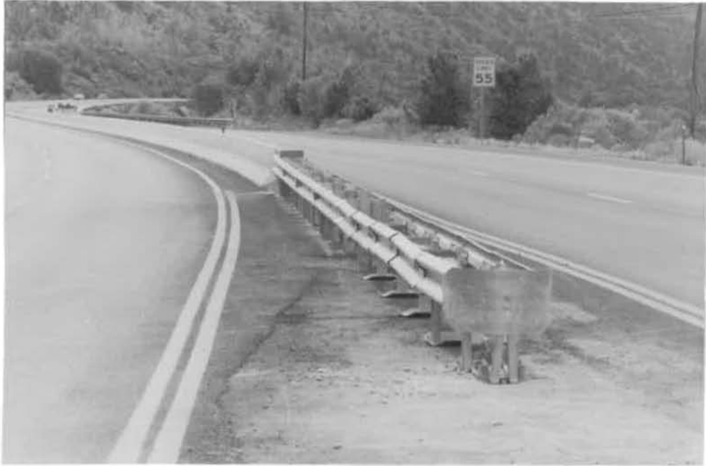
Photo B7. Completed Brakemaster End Terminal.
