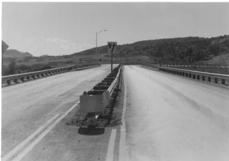
Photo C4. Front view of CAT Terminal.
