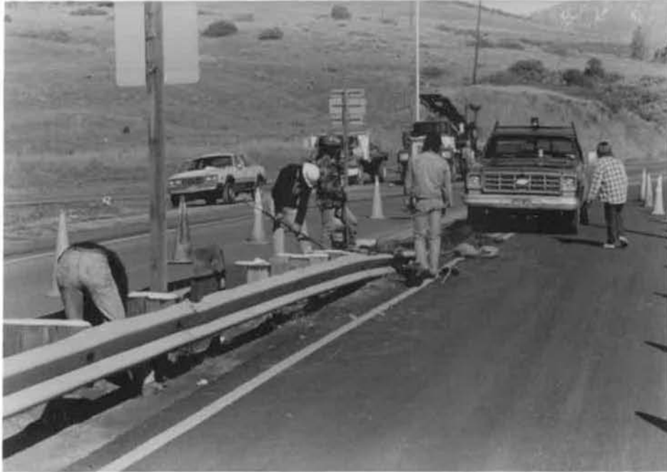
Photo C1. Crew removing old end treatment.
