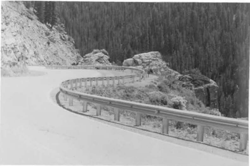
Photo A2. 10-gauge galvanized guardrail on Battle Mountain Pass.
