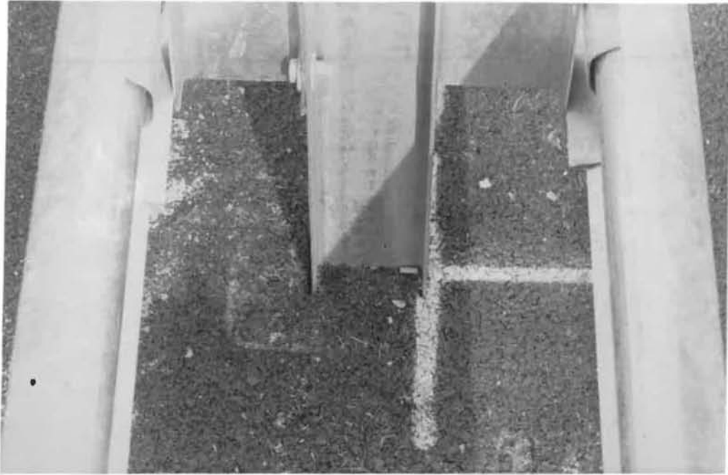
Photo B5. A steel post in the transition section.
