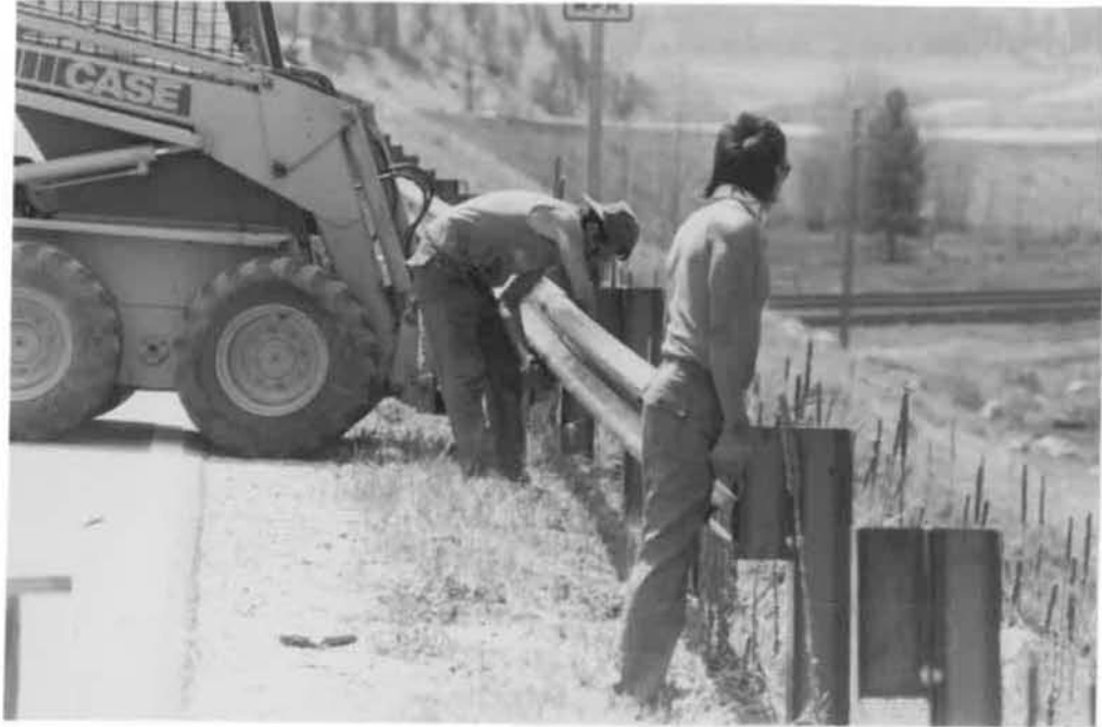
Photo A5. Two men positioning a guardrail panel for installation.
