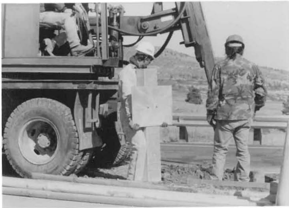
Photo C2. Vertical soil plate and sleeve that is placed over wooden post.
