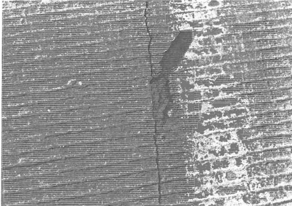
Photograph 7: Plastic parting strip on I-25
