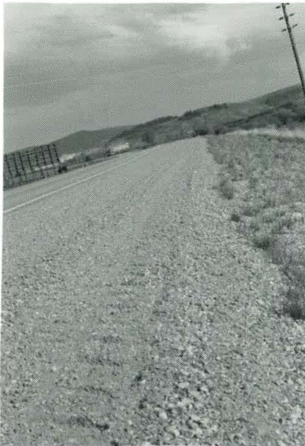
Photo 9 - Shouldering material in good condition on SH-40.
