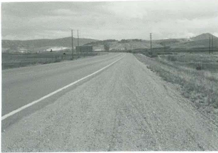
Photo 7 - Completed gravel shoulder on SH-40 near the town of Granby.
