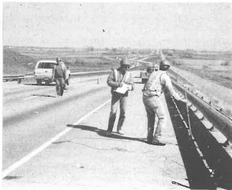
Research staff performing tests of a bridge deck protective system.
