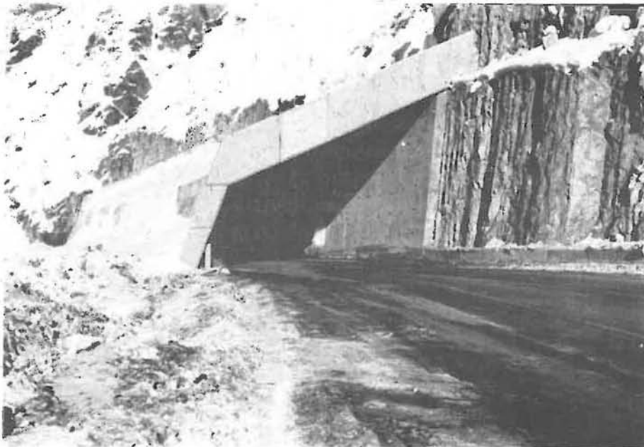
This snowshed, north of Durango is being monitored for avalanche activity.
