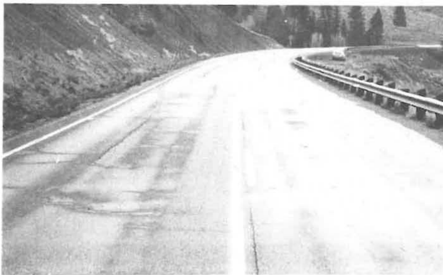
On the right is a polymer-modified asphalt cement. On the left is the standard AC-10F pavement.
