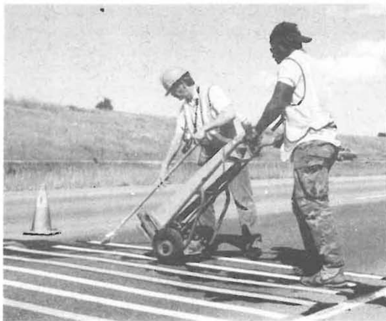
Installation of pavement marking on the test section.
