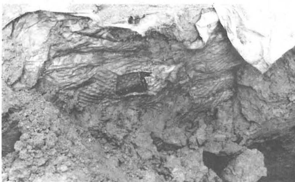
A portion of this curtain drain has been cut in order to evaluate it's effectiveness.
