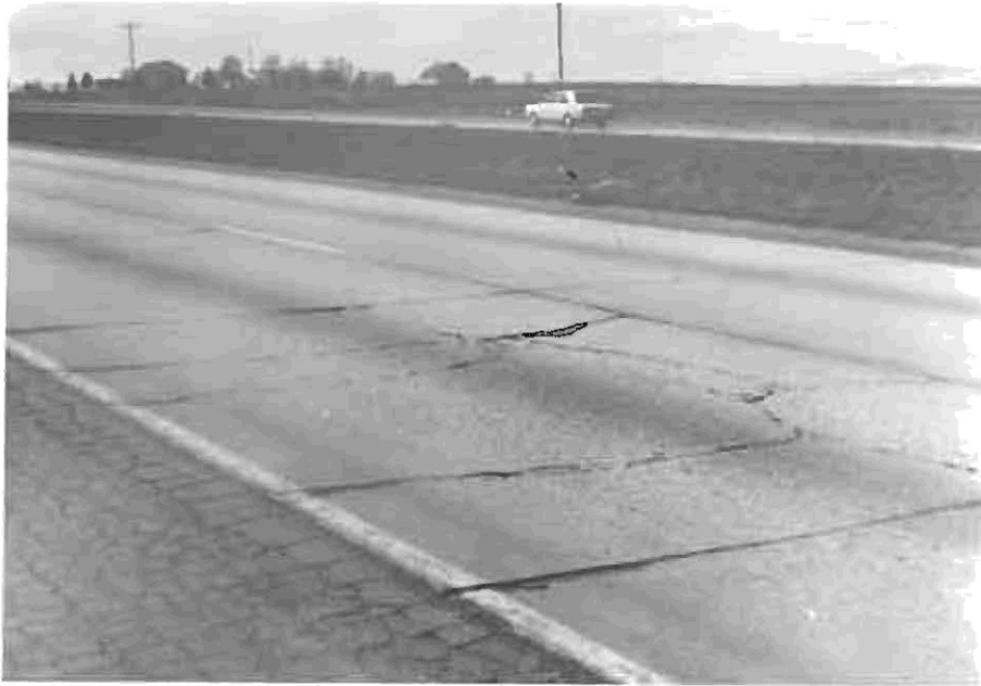
Photo 1: A typical slab that required removal
