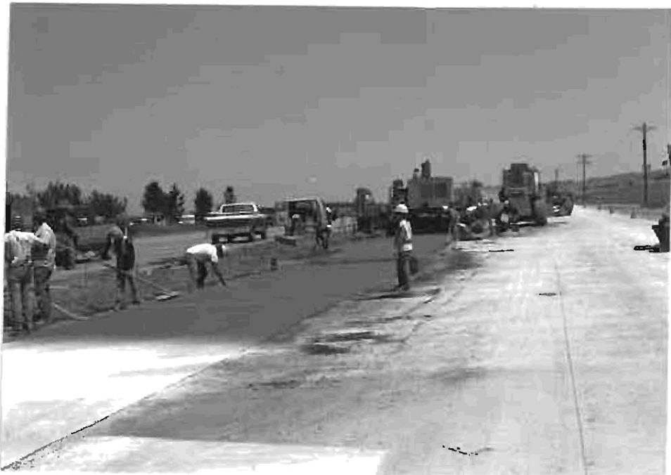
Photograph 3 & 4: The dense graded mixture required more finishing effort than the standard mixture
