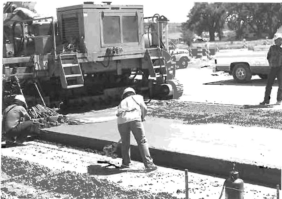
Photograph 1 & 2: A 16 foot inside lane was constructed using dense graded mixture
