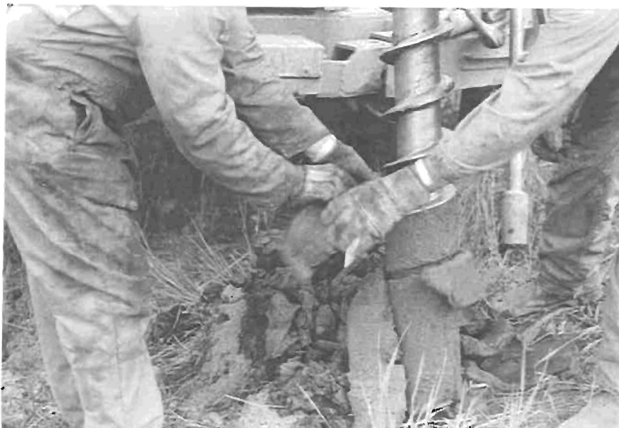
Figure 18 The cohesiveness of the clay was demonstrated by the way strips of mud were peeled off the auger during the installation of the monitoring wells.
