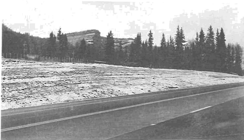
Figure 2 The curtain drains were placed within this hill on the west side of US 550 south of the Purgatory Ski Area.
