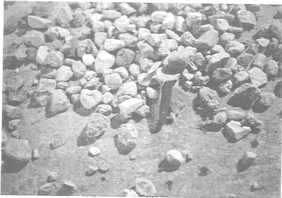
Photo 8 - The granular material placed.
