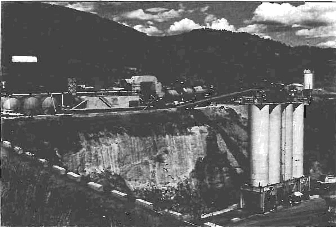
Fig. 3. The Plant Used to Produce HMA for 6th Avenue.
