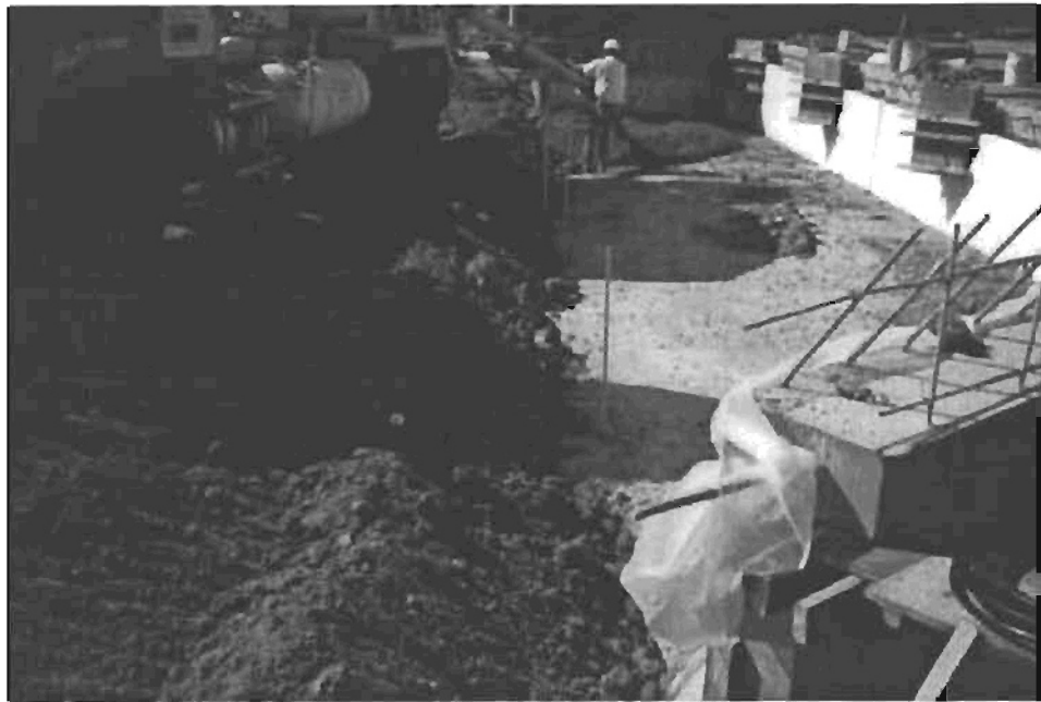
Photo 2: Placement of Flow Fill Behind of Abutment
