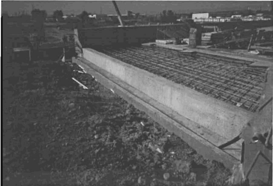
Photo 3: Reinforced Concrete Approach Slab and Sleeper
