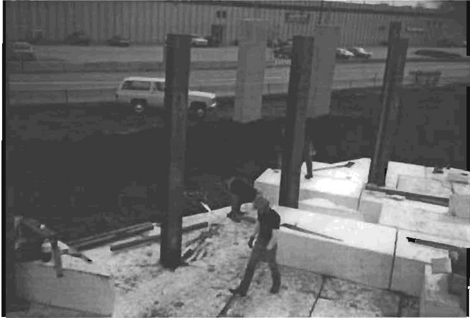
Photo 1: EPS Construction on West Bridge Abutment Approach
