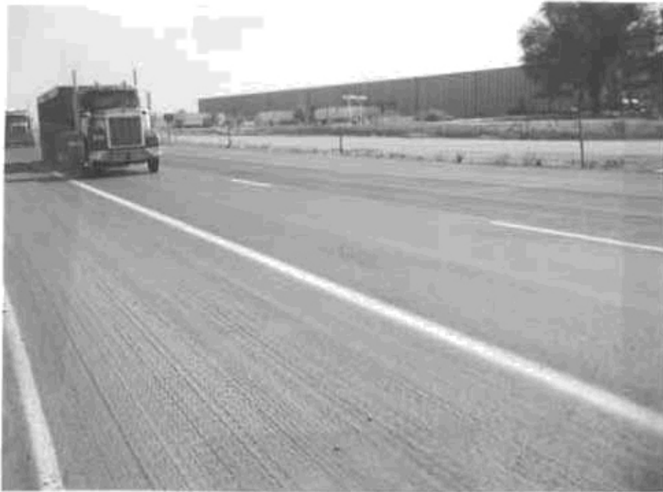
Figure 10. Appearance of Surface After Milling and Base Course Placement.
