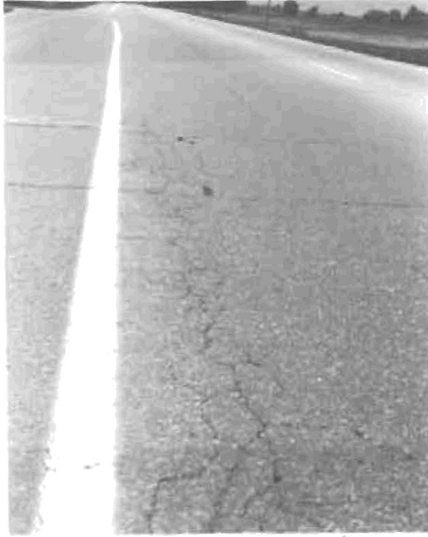
Figure 3. Overview of Existing Pavement Condition Prior to Construction.
