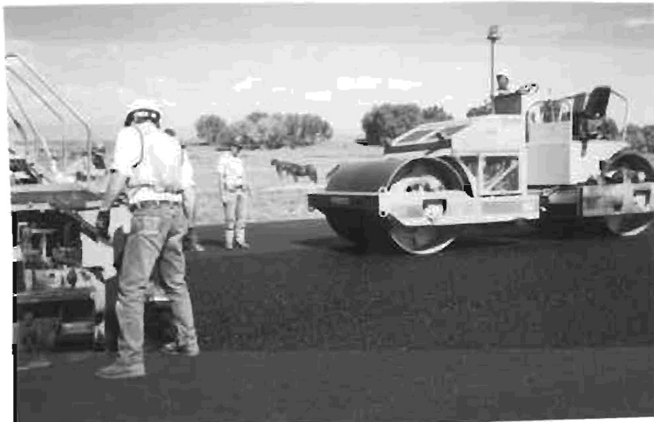
Figure 13. The Breakdown Roller Was Kept Close to the Laydown Machine.
