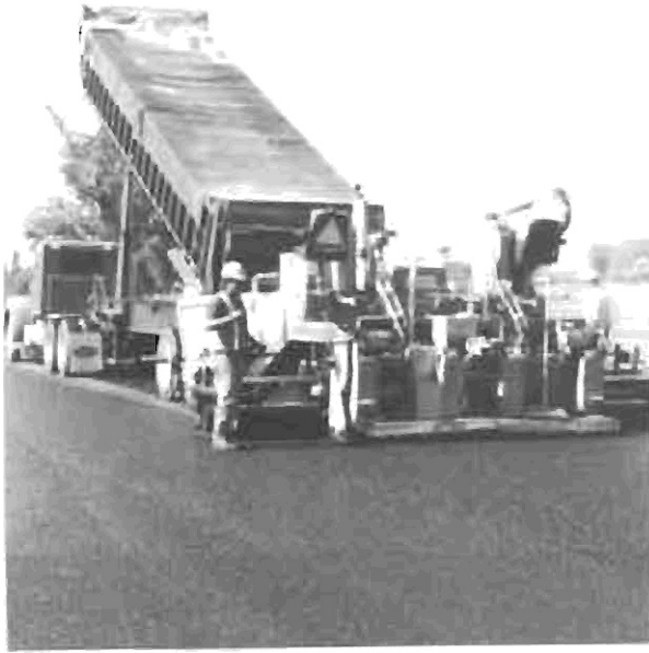
Figure 12. Typical Laydown Operation.
