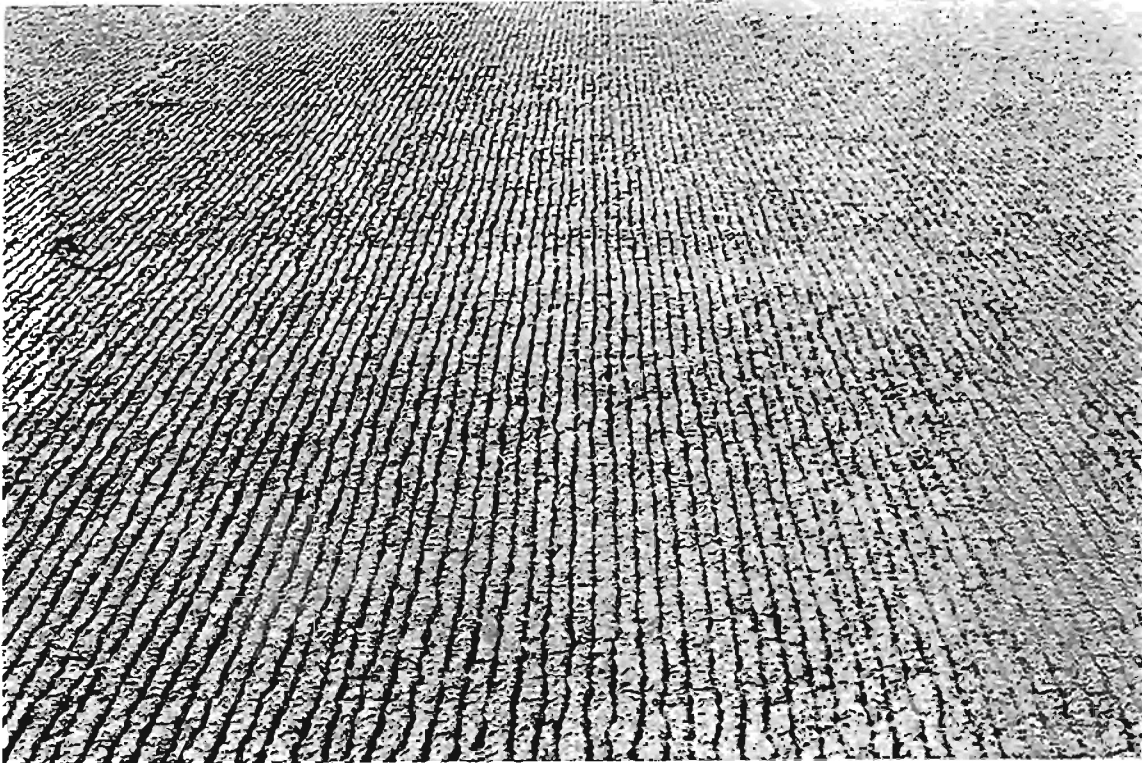
Photo 11: 1/2" uniform spaced transverse tining
