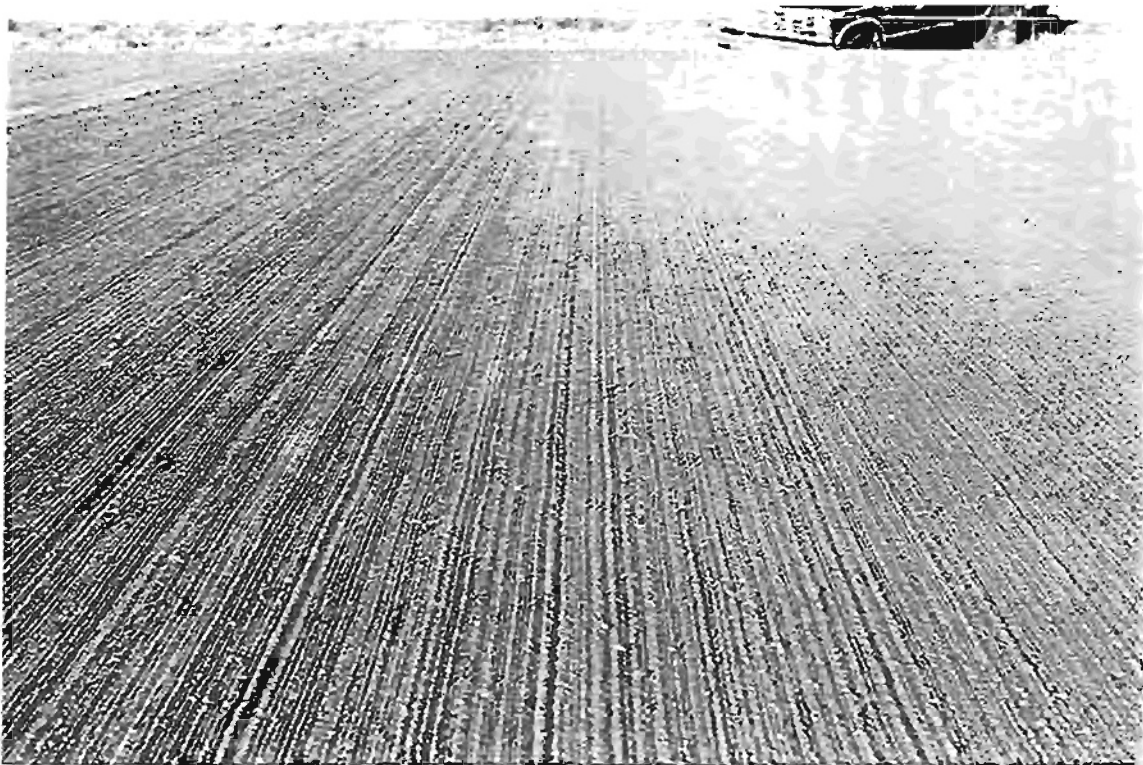
Photo 7 & 8: Installation and close-up view of transverse astro-turf texture
