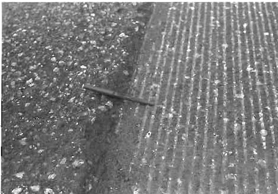
Photo 2 - Planning was performed to a depth of \frac{3}{4} of an inch.
