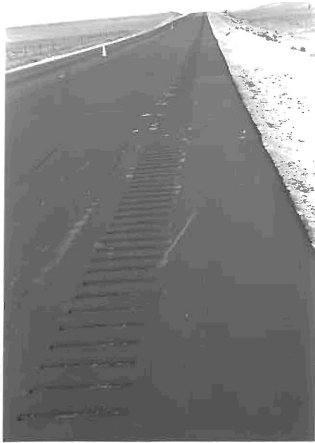
Photo 11- Finished rumble strip on SH-14.
