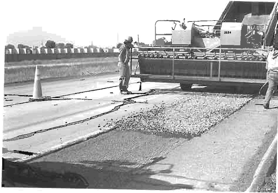
Photo 5 - The cover coat material was placed at 45 lbs./sq.yd.
