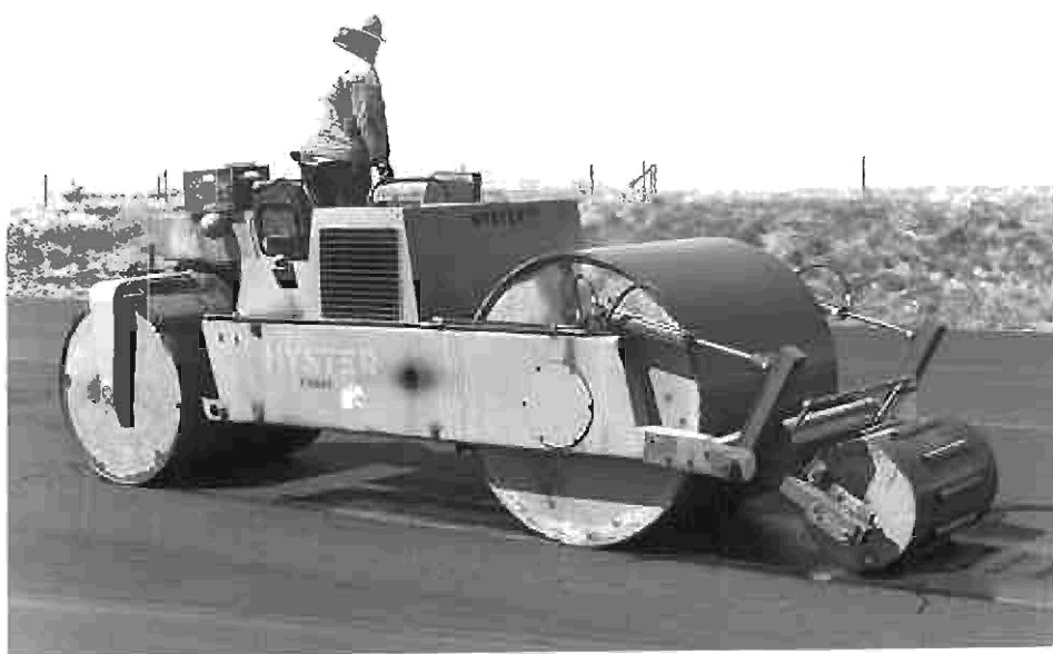
Photo 13 - Rumble strips being placed on SH-63 south of Akron.
