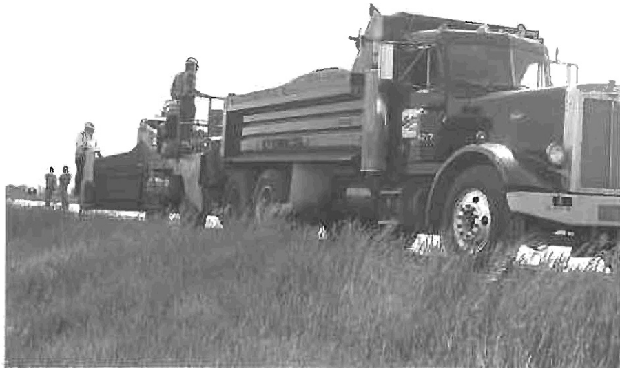
Photo 4 - Placement of the aggregate for the chip seal.
