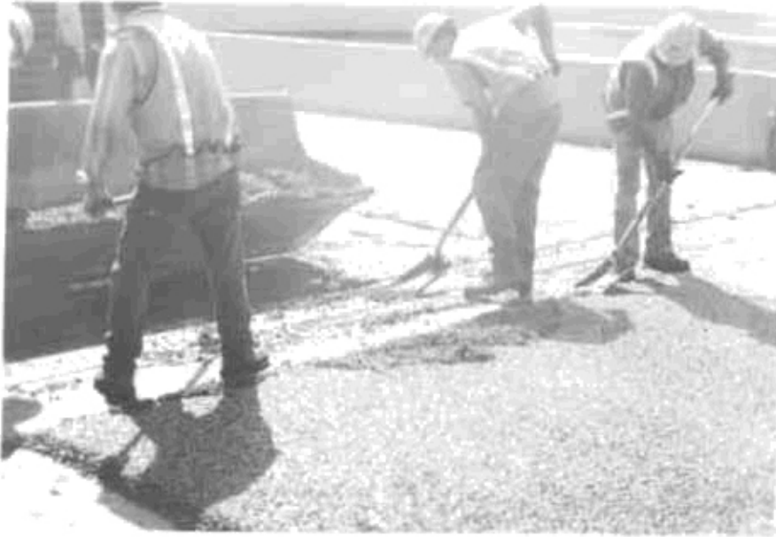
Figure 9. Hand work is required at the expansion joint.
