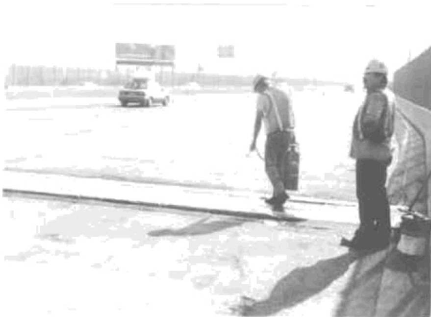
Figure 8. Preparing the joint prior to SMA placement.
