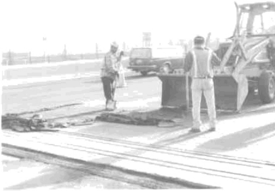
Figure 7. Removing the taper at the expansion joint.
