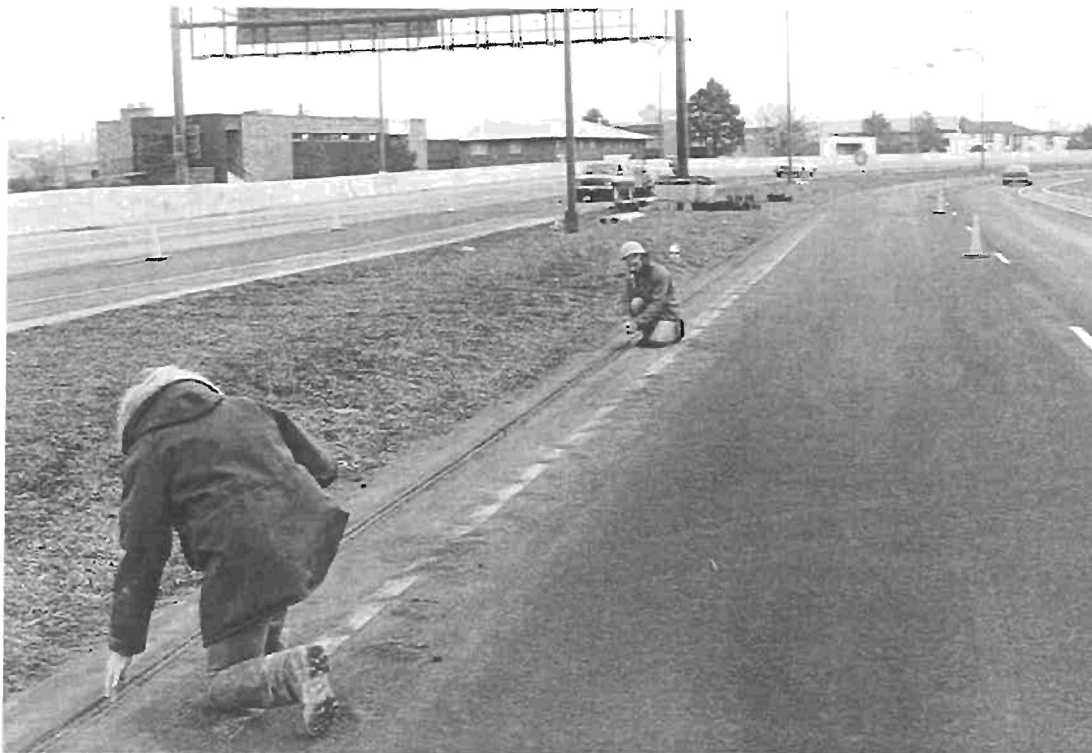
Laying out the Guide lines
