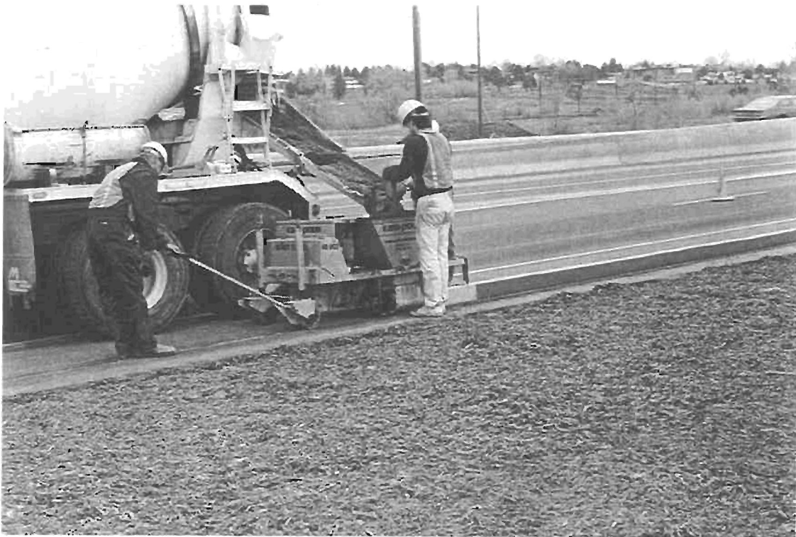
The Curb slip form machine
