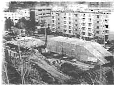
JR Embankment No. 1 at Completion (Background)
