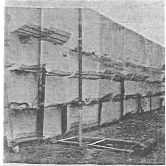
Wall Under Construction (a)
