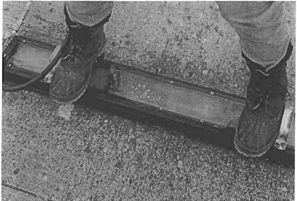
Figure 5 The drops in the center of the chamber show a severe leak. The air flow through the failure can't bubble; it just sprays the solution on the bottom of the window. This can also happen if the vacuum level in the chamber is too high with a smaller leak.
