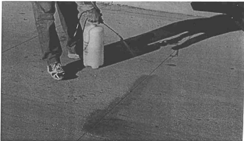
Figure 2 Wet the joint and the pavement surface for about 4" on each side.
