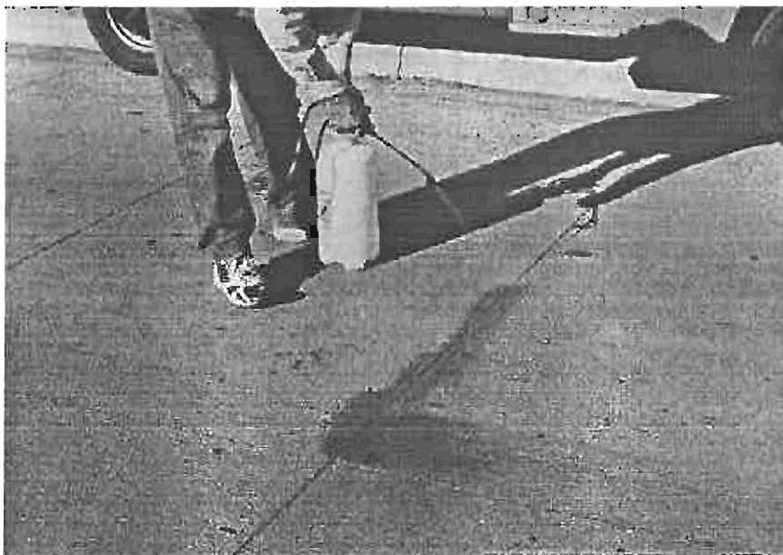
Figure 5 The joint to be tested and the pavement surface where the test chamber will sit are sprayed with a soapy water solution. It is important to wet the joint thoroughly.
