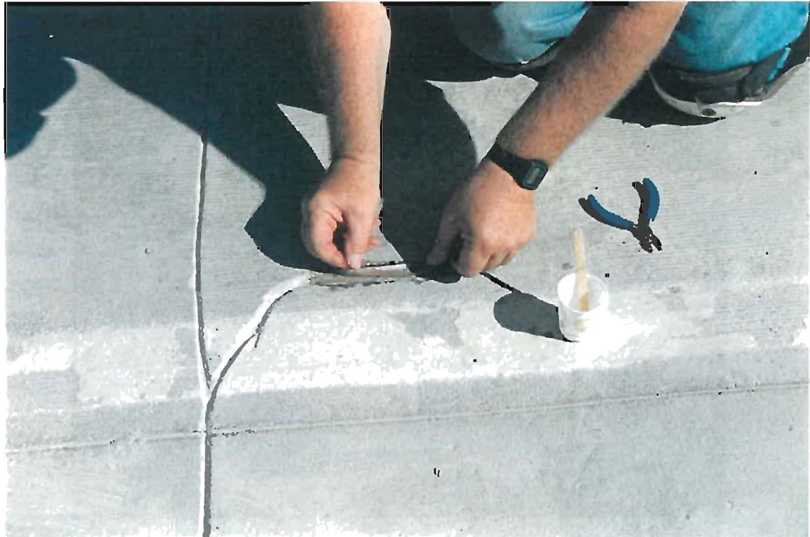
Figure B.10 - Installing Concrete Surface Gages at CDOT Project #2
