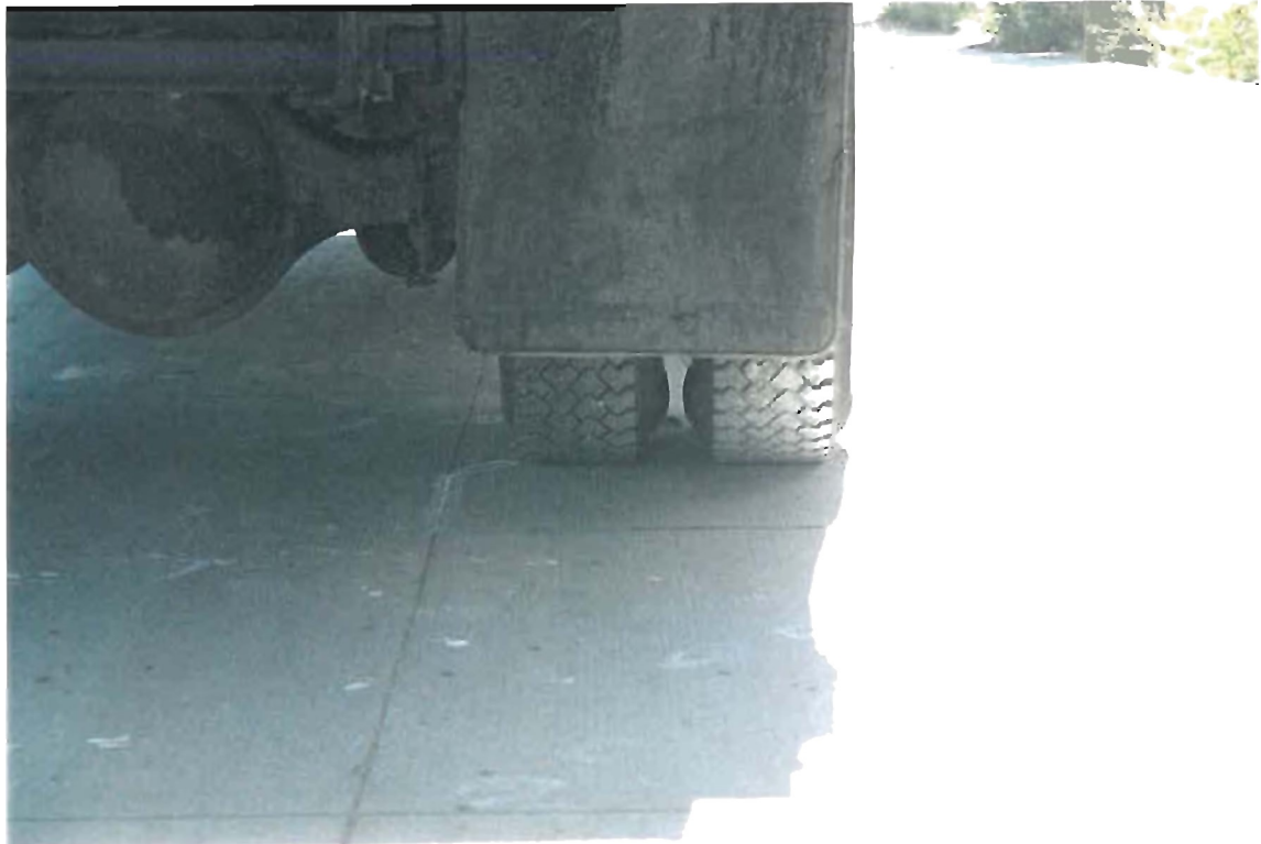
Figure A.9 - Typical Placement of Truck Tires Adjacent to Strain Gages for Load Testing
