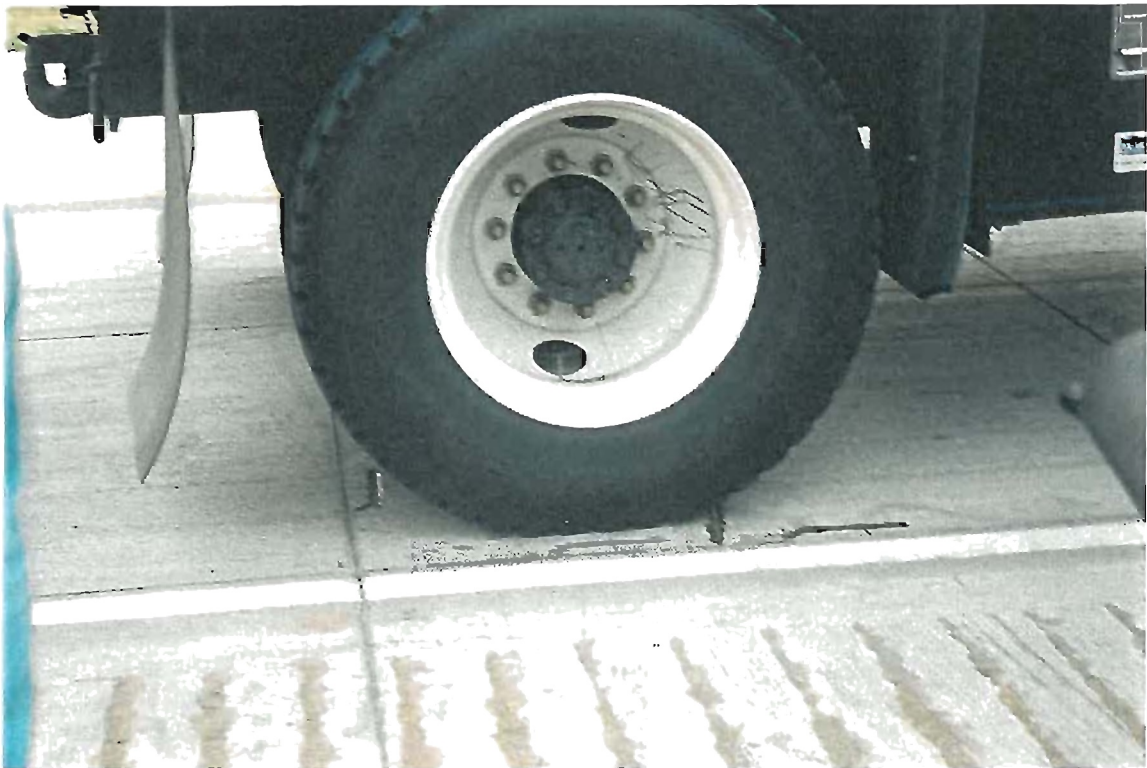
Figure C.6 - Typical Placement of Truck Tires Adjacent to Strain Gages for Load Testing
