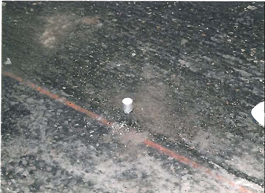
Figure B.8 - Installed Invar Reference Rod Prior to Paving
