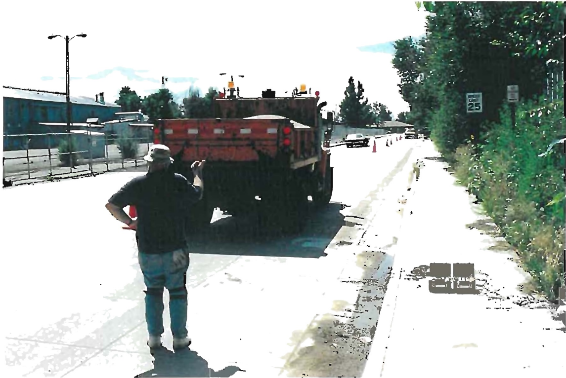
Figure A.8 - Load Testing at CDOT Project #1
