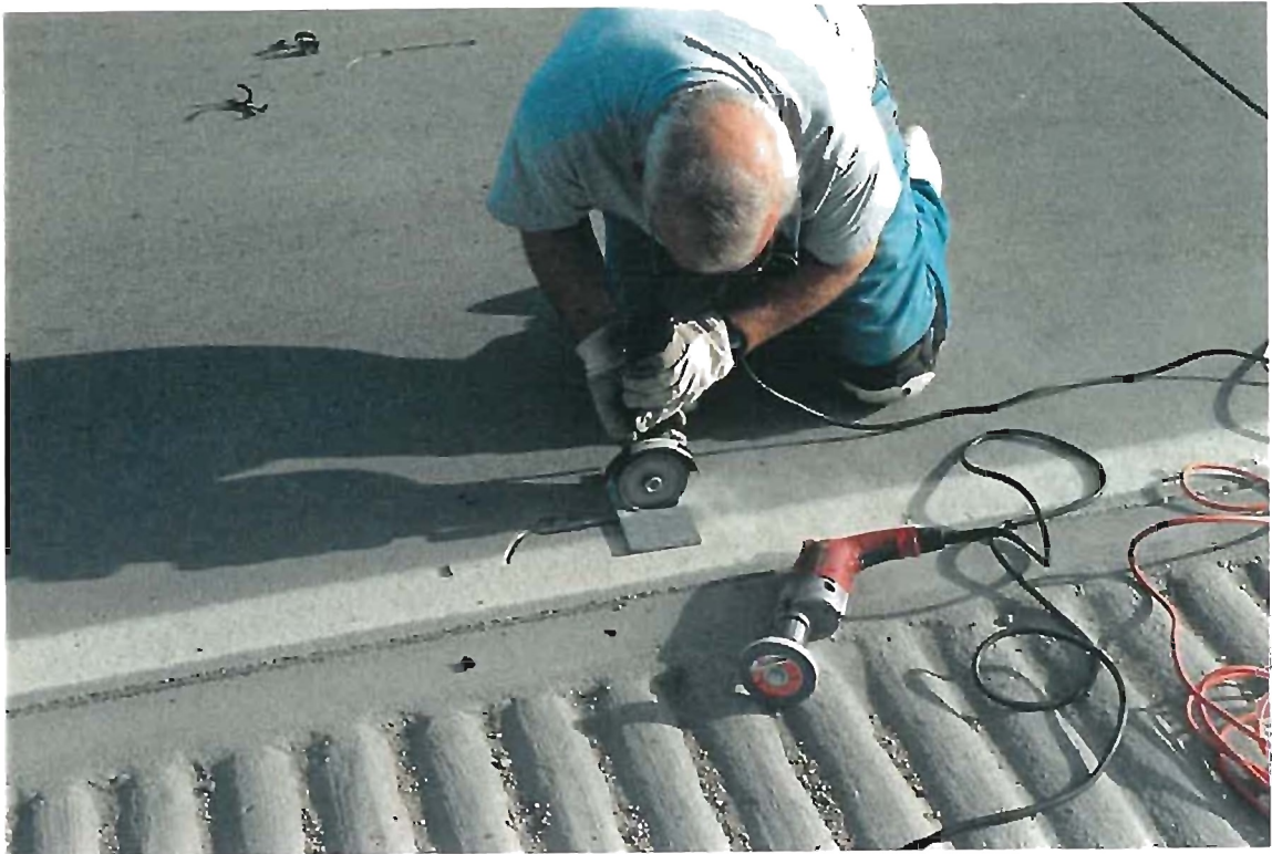
Figure B.9 - Preparing Concrete Surface for Strain Gages at CDOT Project #2
