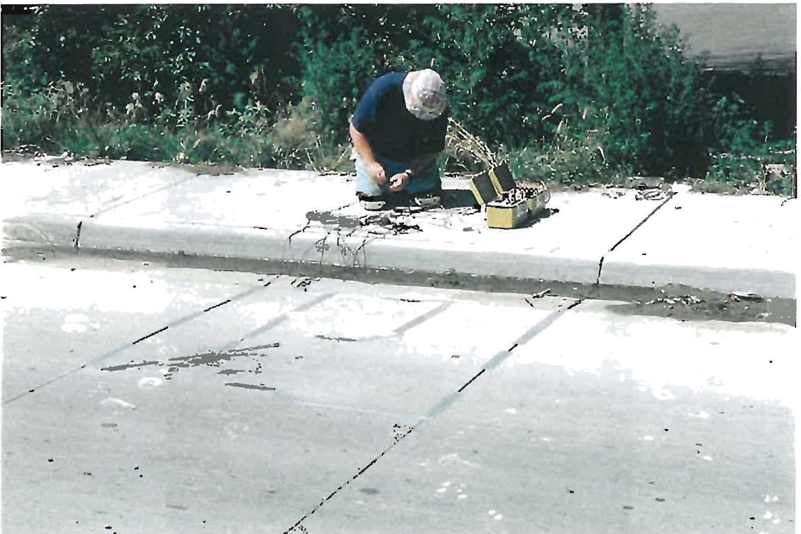
Figure A.7 - Typical Strain Gage Layout and Load Testing Setup at CDOT Project #1
