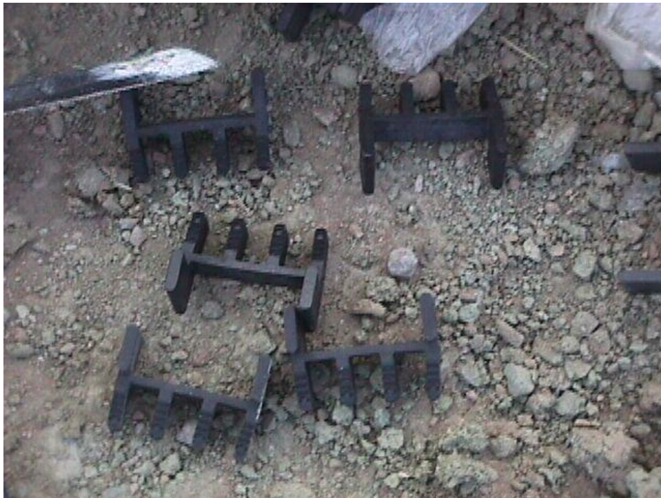
Figure B-10. The Standard Mesa Connectors which provide the positive mechanical connection strength between blocks and between blocks and geogrid. This connector has four “teeth” that fit down into the groove of the block (Fig 8) and two “flags” where the geogrid is hooked. The rear of the cavity of the next row of blocks rests against the two large flags. This provides connection strength between blocks.
