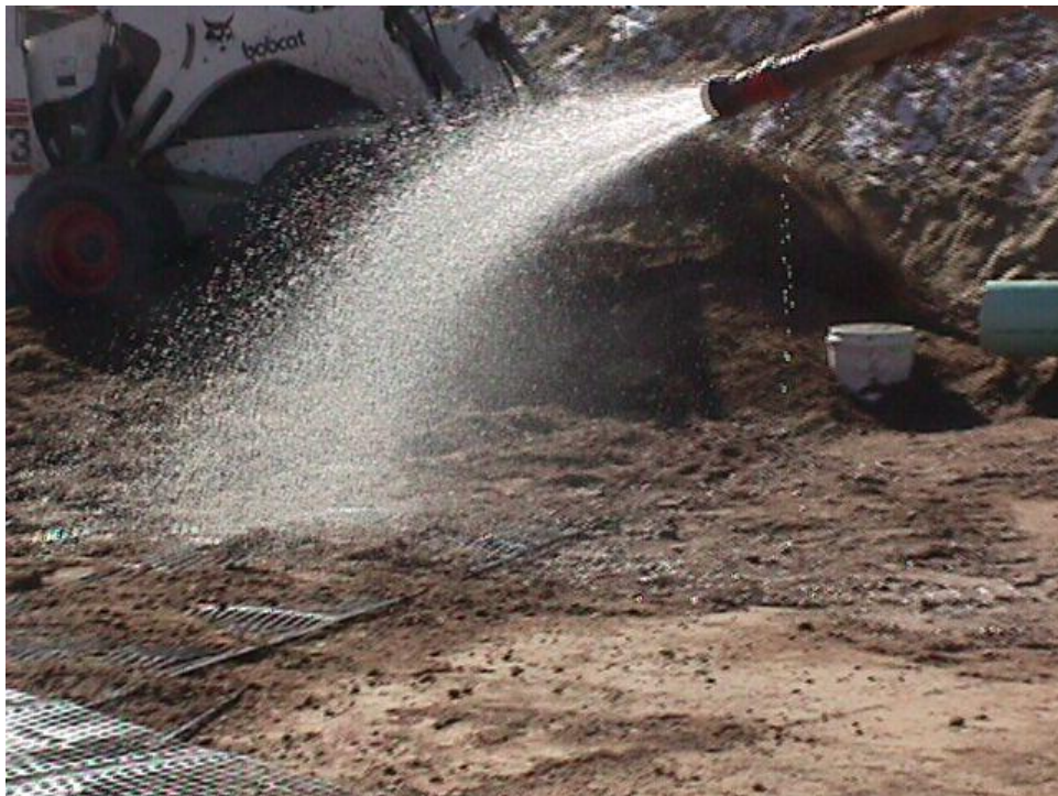
Figure B-14. Water was added before the fill was compacted.
