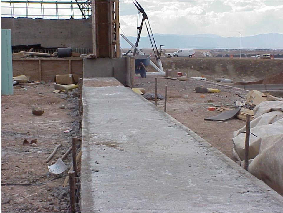
Figure B-37. Leveling pad for the upper MSE wall.
