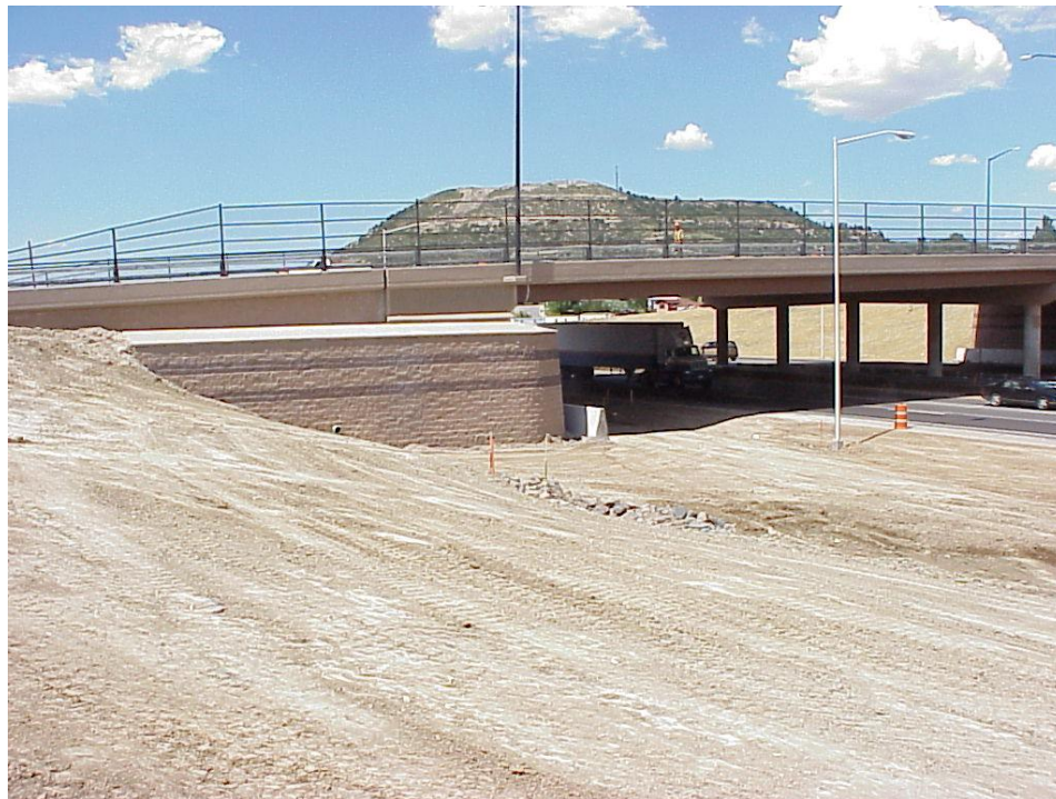
Figure B-3. Southwest view of the completed Founders/Meadows bridge structure.
