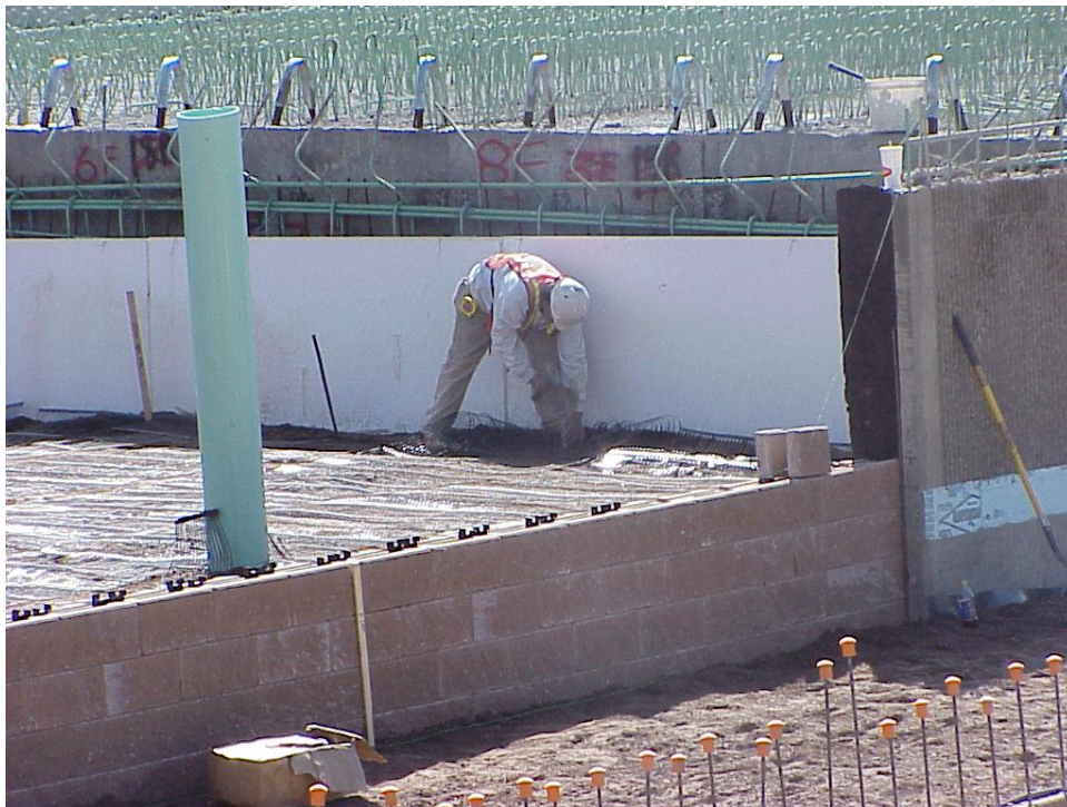
Figure B-36. The wrapped geogrid behind the abutment wall.
