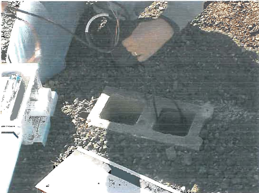
Figure 19. Installation of sensors and close-up of storage block.
