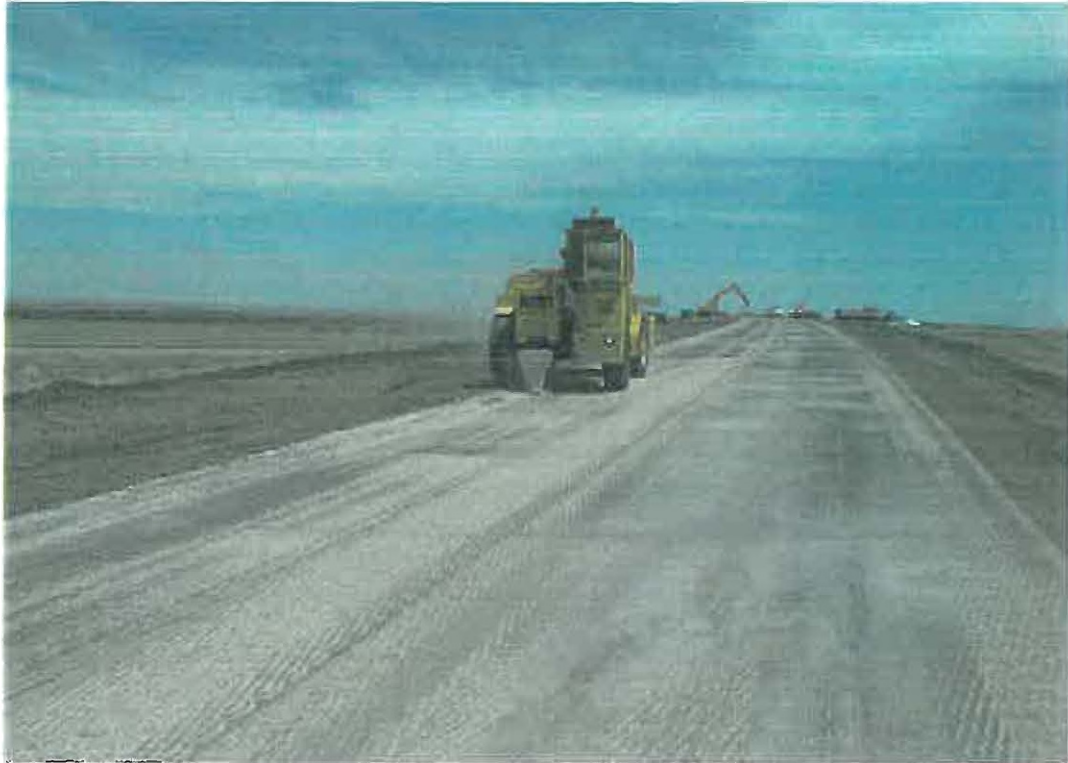
Figure 9. Resonant treatment process.
