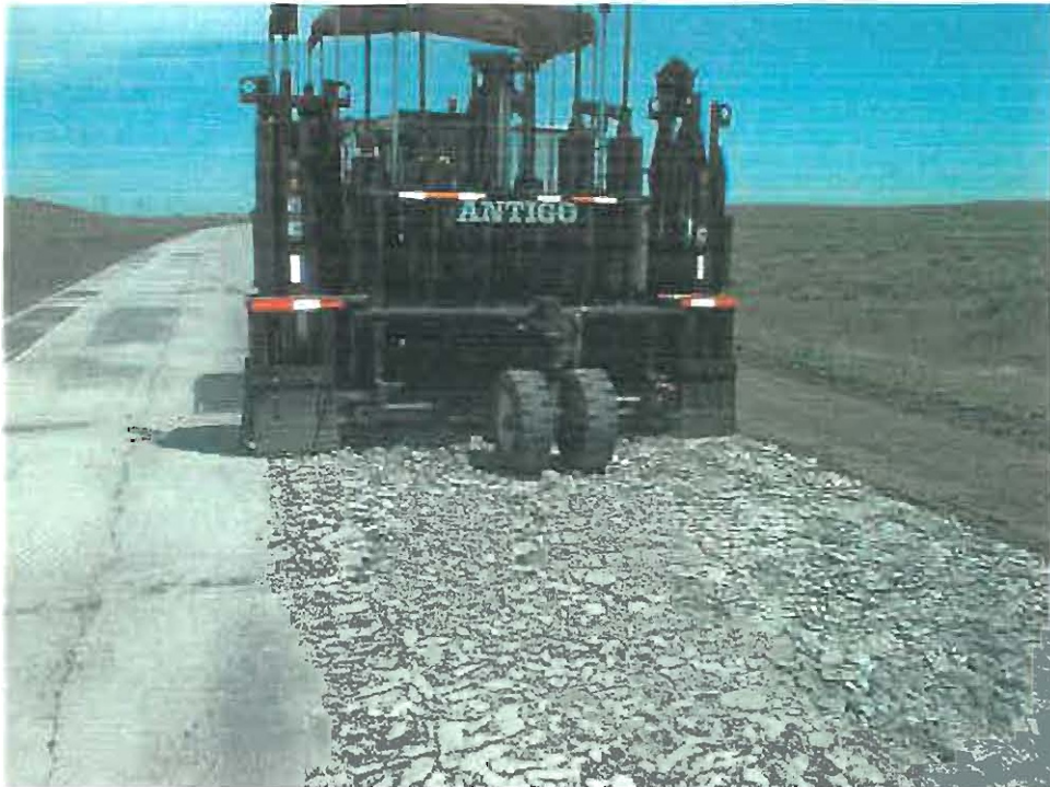
Figure 11. Multi-head hammer in action.
