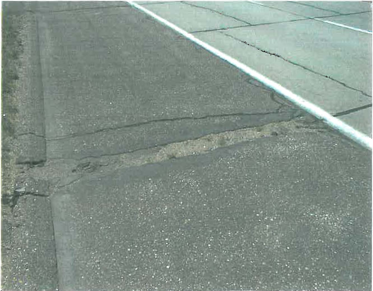
Figure 7. Condition of shoulder before being broken up by the Bomag.
