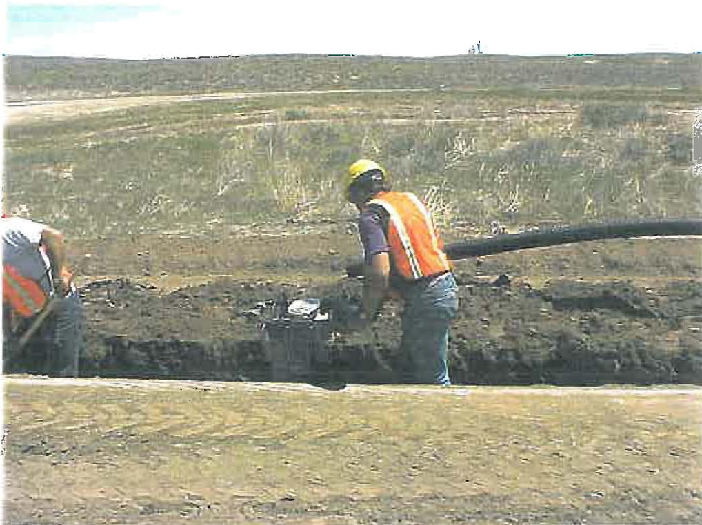
Figure 14. Preparation of trench for edge drain installation.
