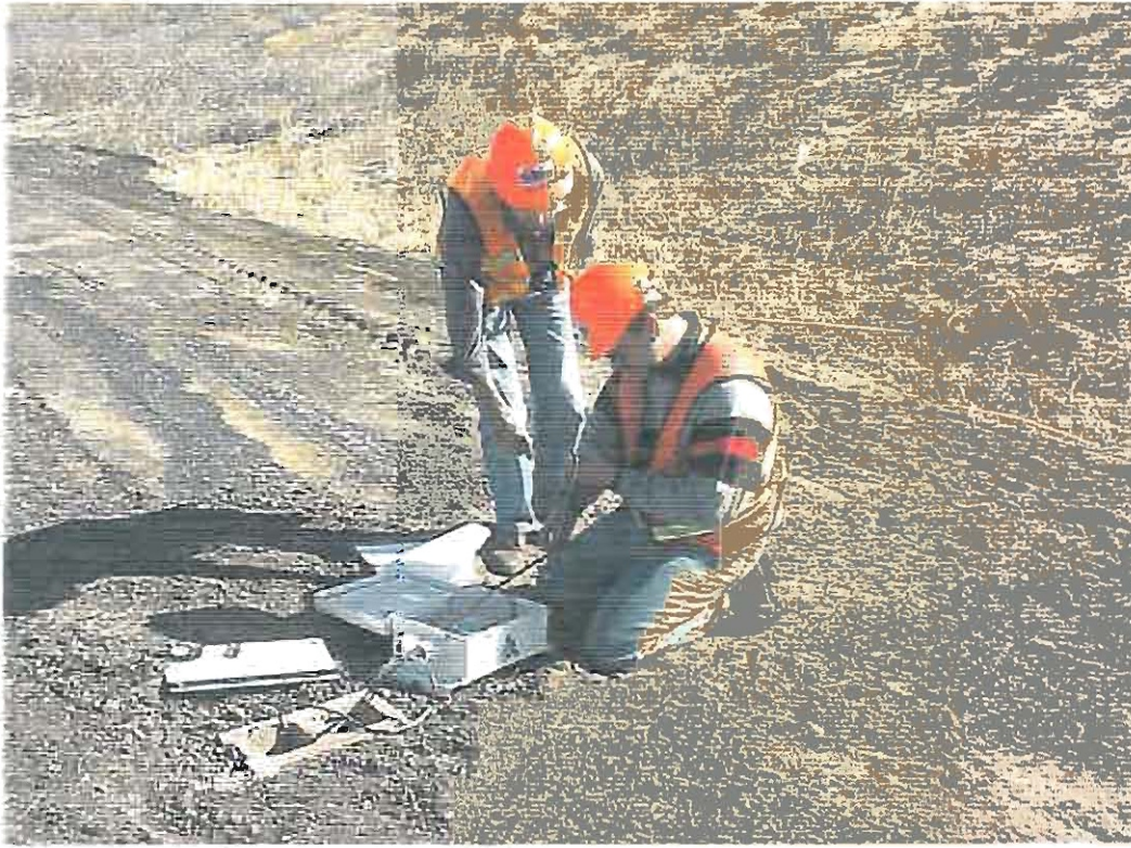
Figure 18. Installation of the moisture sensors.
