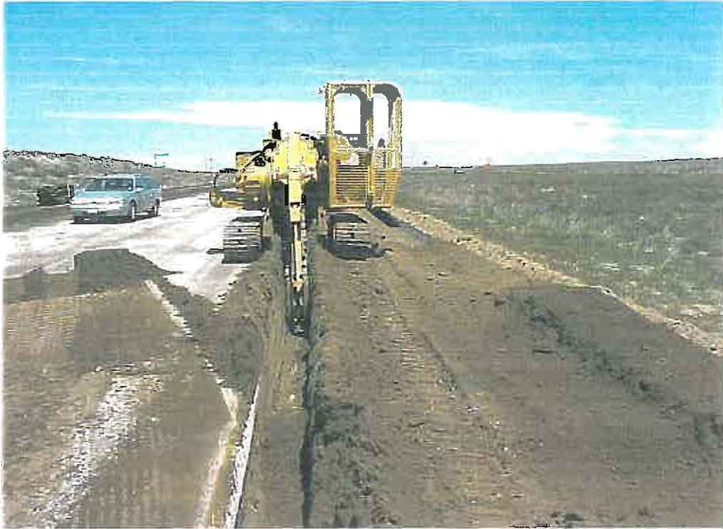
Figure 13. Trencher used for installing edge drain.
