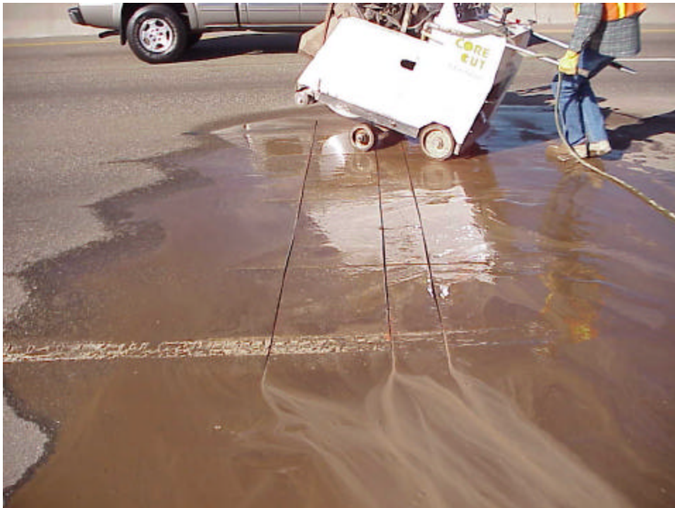
Sawing of the cross section slab. Three saw cuts were made across the lane width. Cross cuts were made to break the slab into four pieces.
