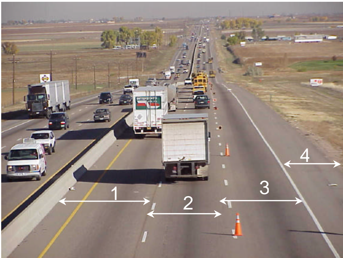
Figure 6 Paving Construction Sequence
