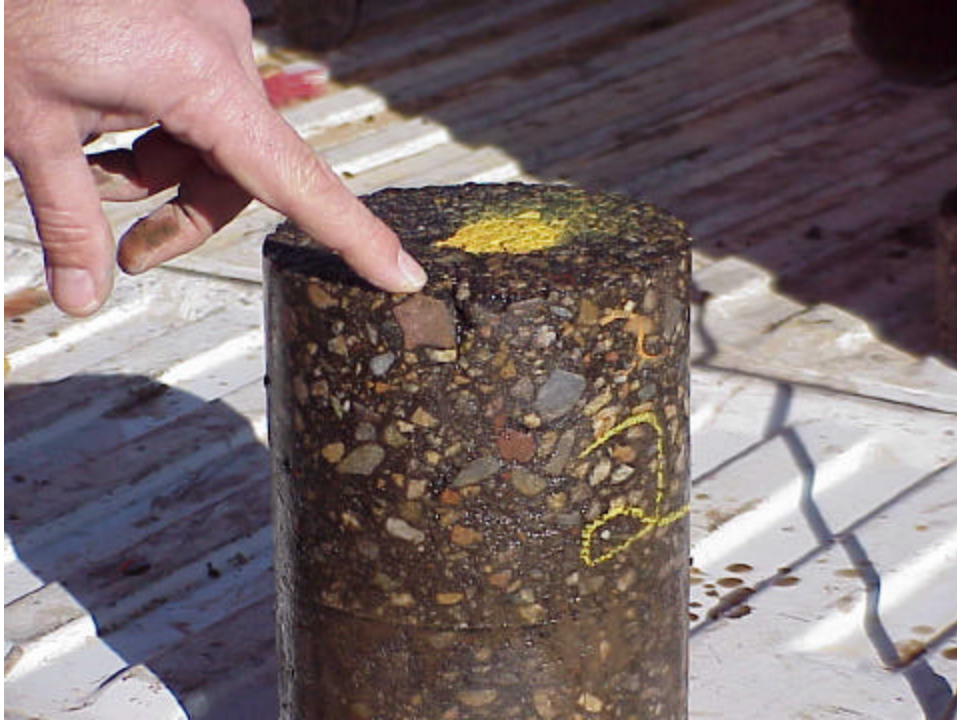
Freshly cut, wet core showing aggregate skeleton. This is Core # 2 shown in the core location figure. It was taken at the end of a short longitudinal crack.
