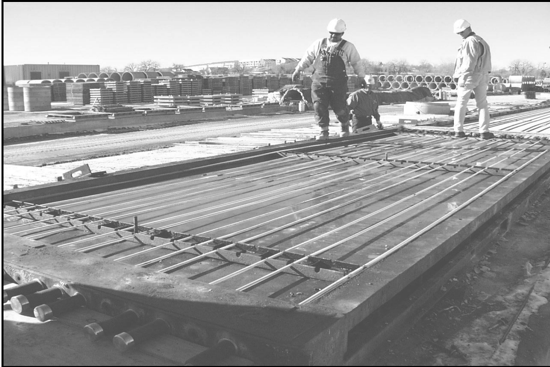
Figure 4.2 FRP prestressed panel construction
