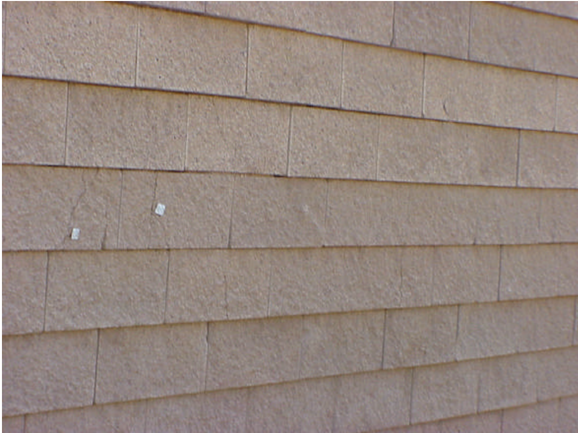
Photo 8. Cracks in the Lower Part of the Abutment.
