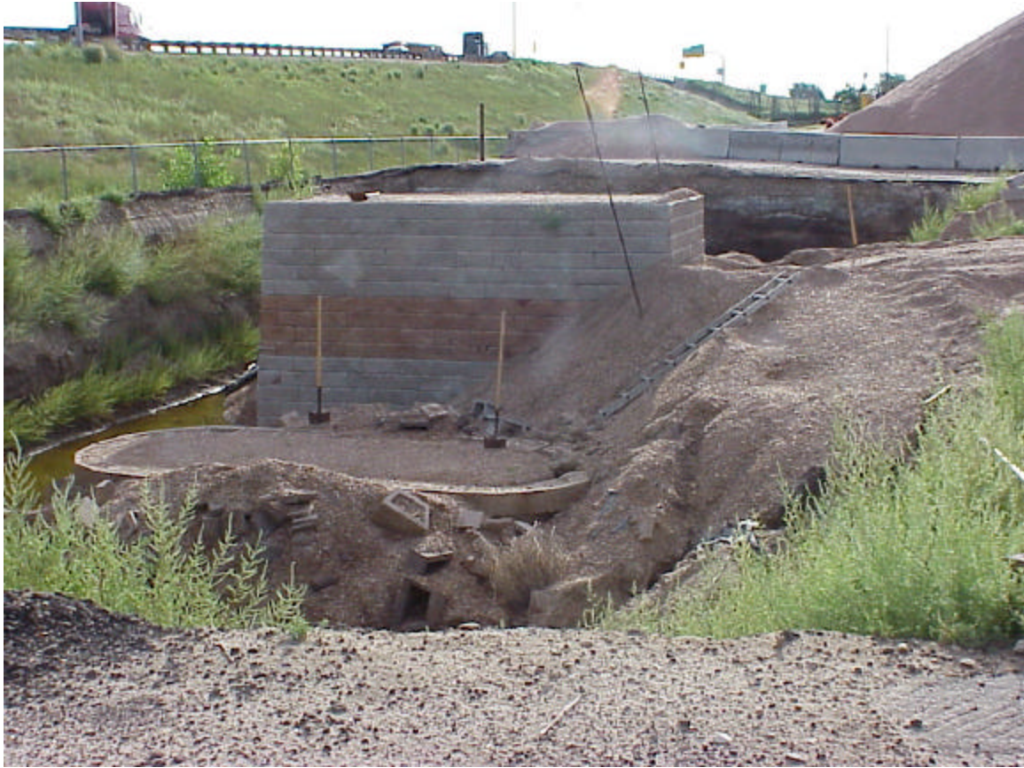
Photo 9. Dismantling Operation of the Havana Maintenance Structures.
