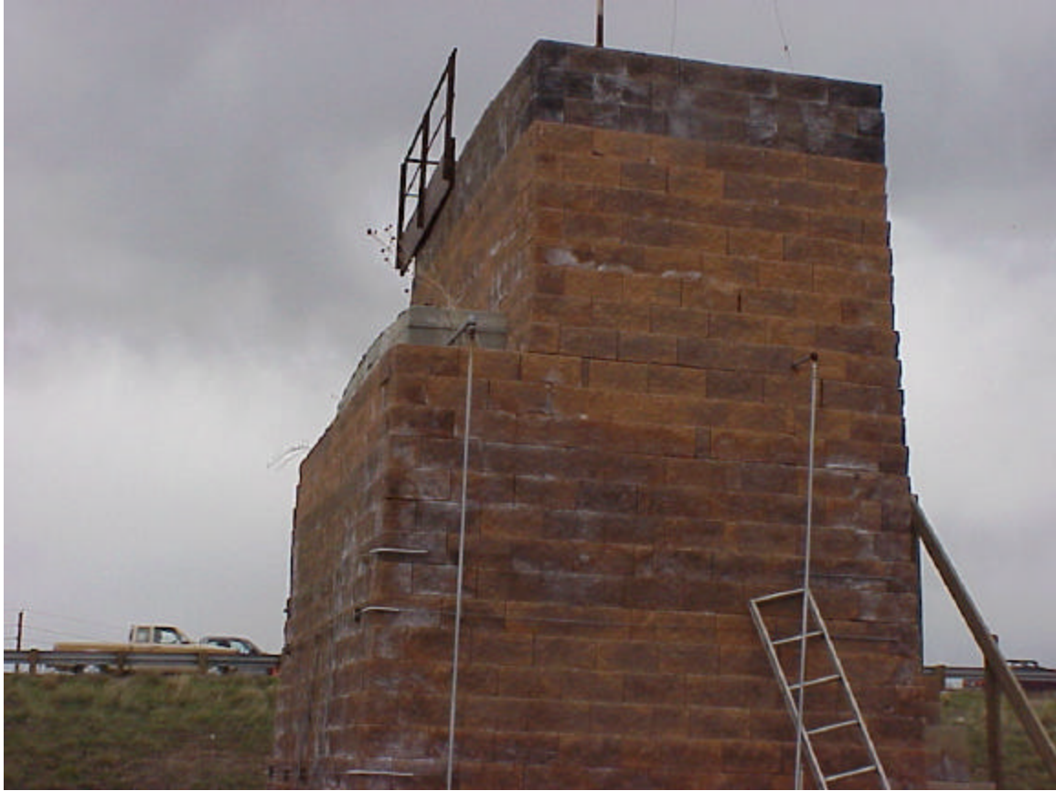
Photo 2. Upper Portion of the Abutment Structure.
