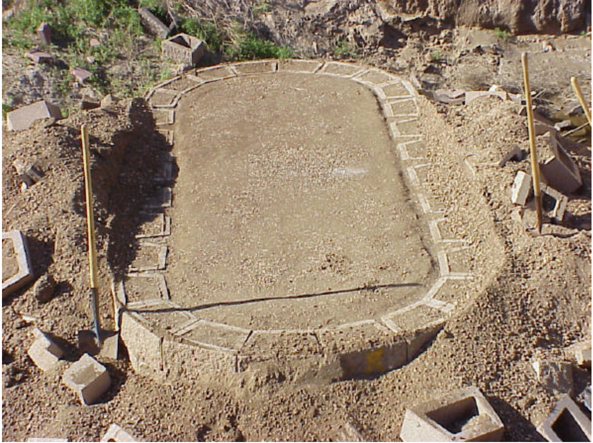
Photo 10. Dismantling in Progress: The Outer Pier at Row 10 from bottom.
