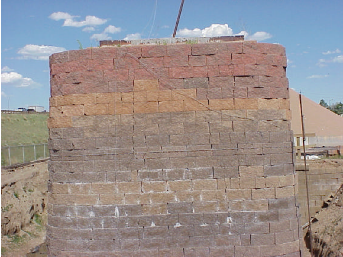
Photo 5. The Outer Pier Structure.
