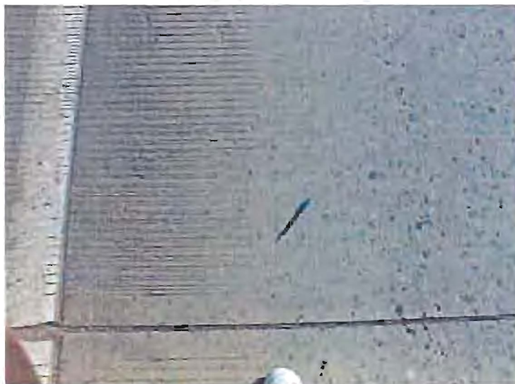
Figure 4. A detailed view of transverse tining at Test Section 1 between mileposts 244.42 and 244.45, east-bound US285. The right-hand ½ of the photograph shows where transverse tining has been ground. The grinding tapers to the left showing remnant transverse tining texture. Note pen for scale.
