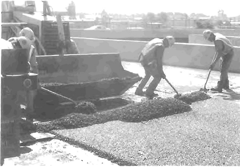
Figure 23. Handwork is required at the expansion joint.
