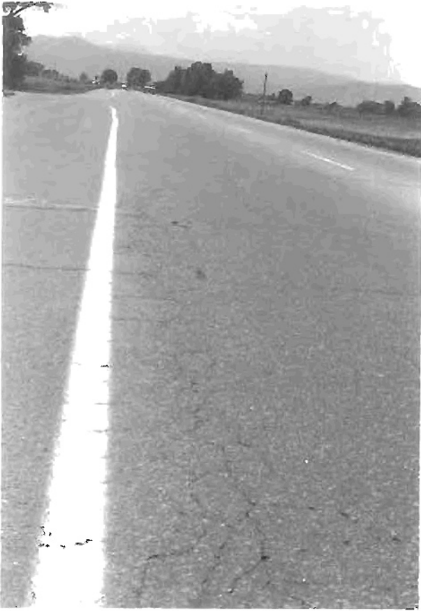
Figure 3. Overview of existing pavement.
