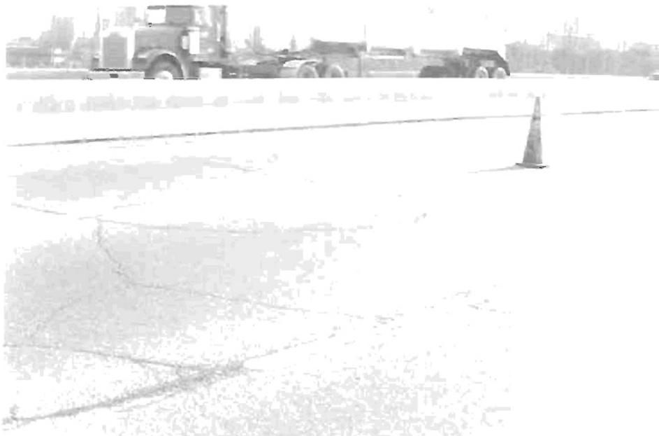
Figure 17. Typical cracking pattern prior to paving.
