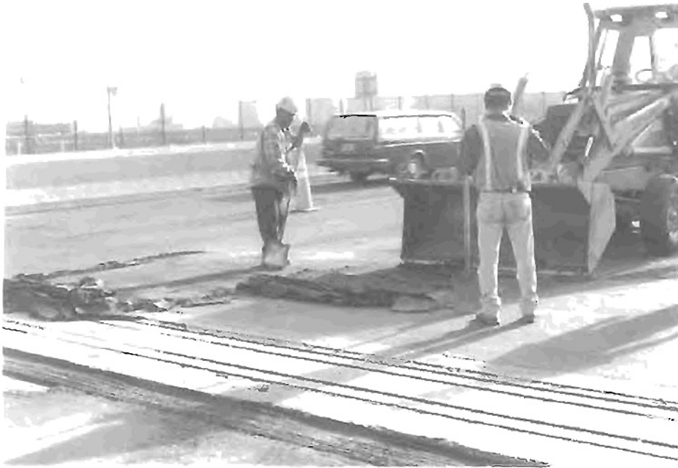
Figure 21. Removing the taper at the expansion joint.
