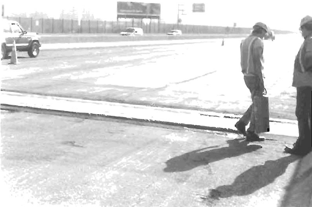
Figure 22. Preparing the joint prior to SMA placement.
