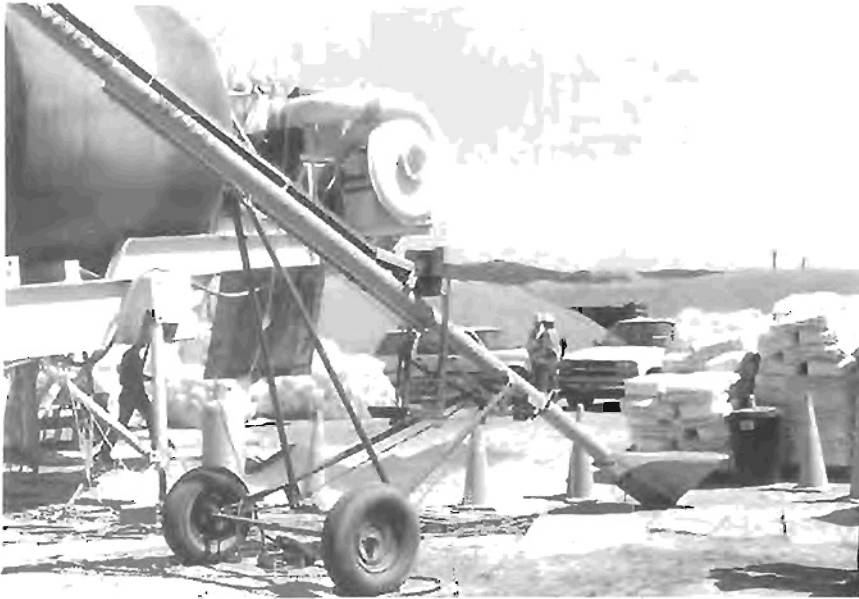
Figure 5. Auger system initially used for Vestoplast S
