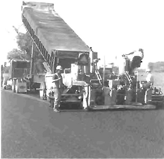
Figure 7. Typical laydown operation
